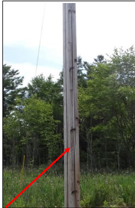
Line V182 Structure 134
