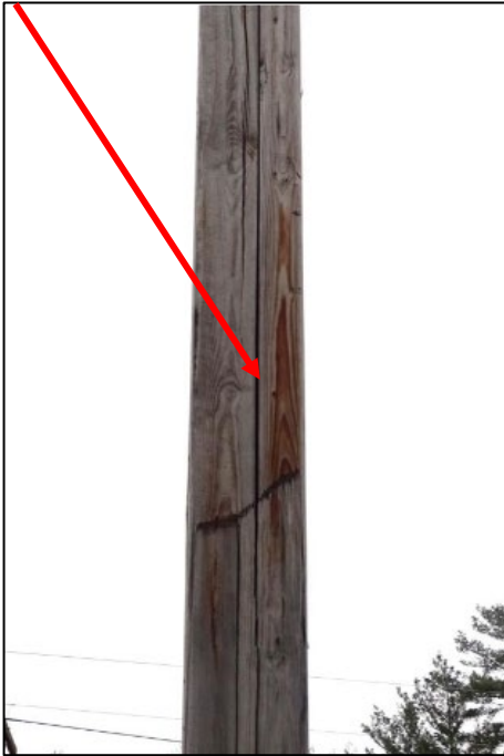
Line C189 Structure 67
