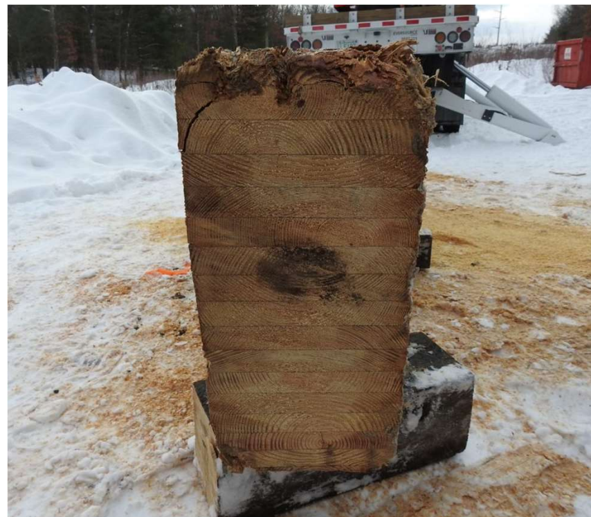
Rotting Cross Section – R187 Line, Structure #7
