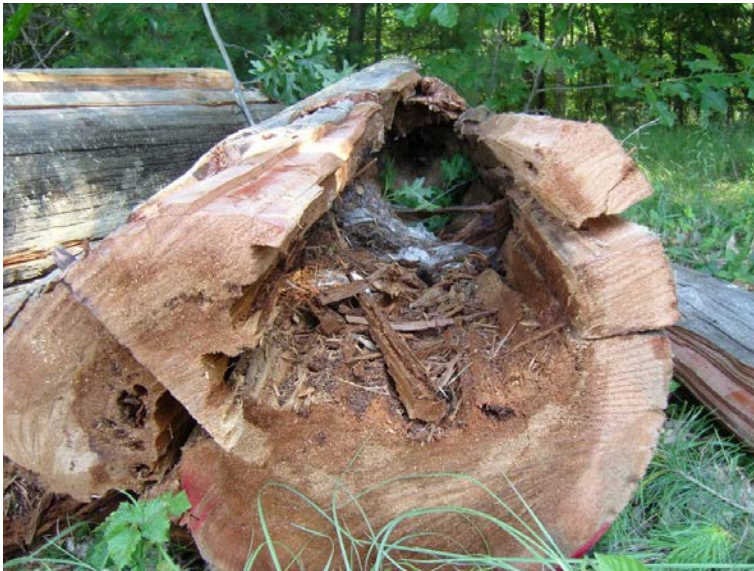
Degree of Woodpecker Damage (this is not a 354 Line structure)
