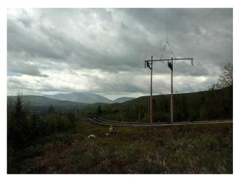
These poles and conduit were replaced in 1986 thus should last until 2060, since the 1948 poles they replaced are still in service.
