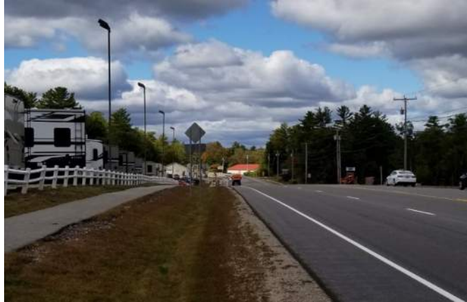
Discrete portions of NH Route 202 in Chichester feature a sidewalk on both sides of the highway, occasionally separated from the roadway by a drainage swale
