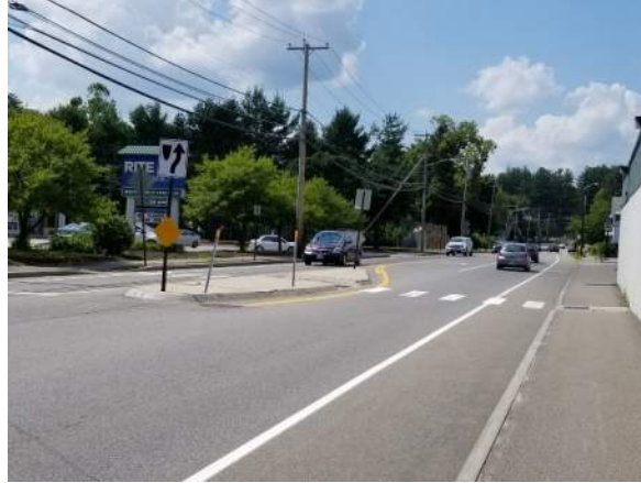
Pedestrian crossing island on North Main Street/Route 3 in Concord
