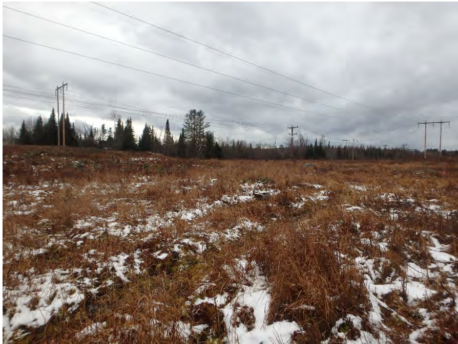
Photo 2. Existing ROW conditions near structure 24. Stantec, November 29, 2016.
