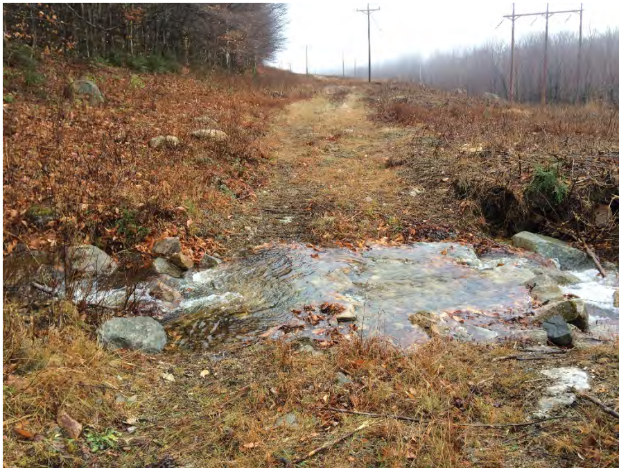
Photo 16. Existing ROW conditions near structure 205. Stantec, November 16, 2016.
