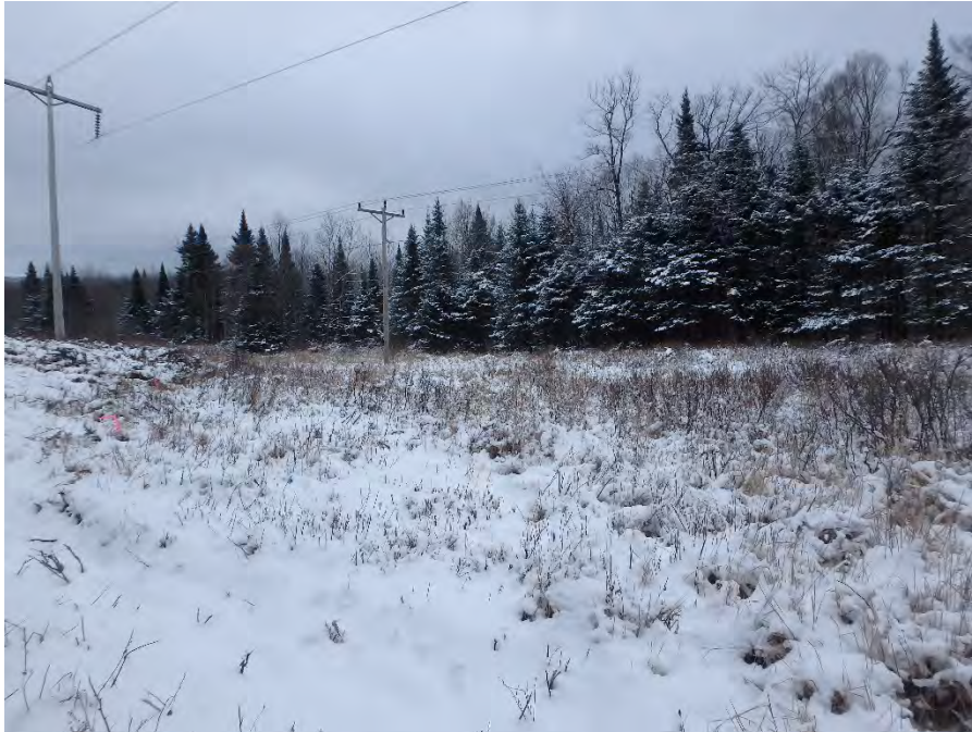
Photo 11. Existing ROW conditions near structure 172. Stantec, December 6, 2016.
