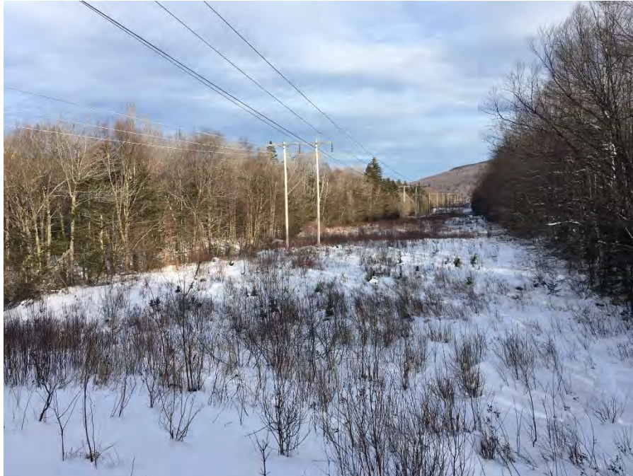
Photo 9. Existing ROW conditions near structure 160. Stantec, January 24, 2019.
