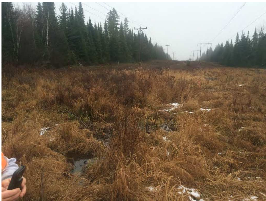
Photo 6. Existing ROW conditions near structure 36. Stantec, November 30, 2016.
