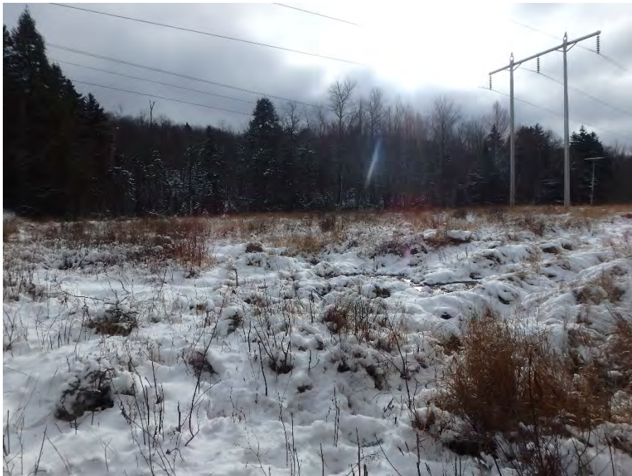
Photo 12. Existing ROW conditions at structure 178. Stantec, December 6, 2016.
