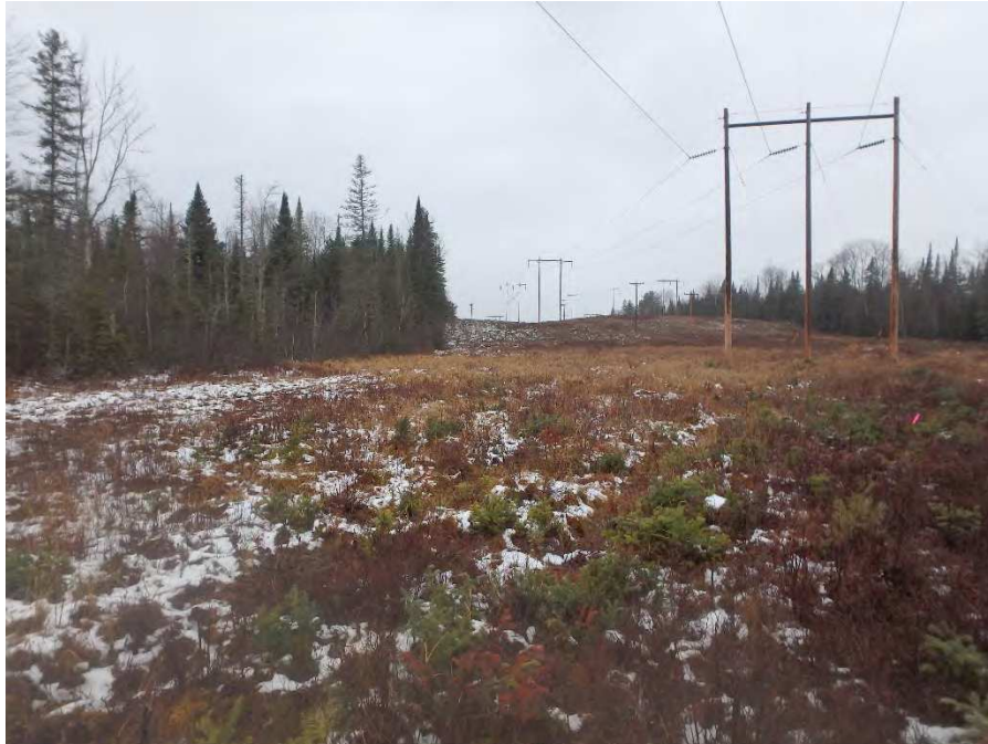
Photo 5. Existing ROW conditions near structure 33. Stantec, November 29, 2016.
