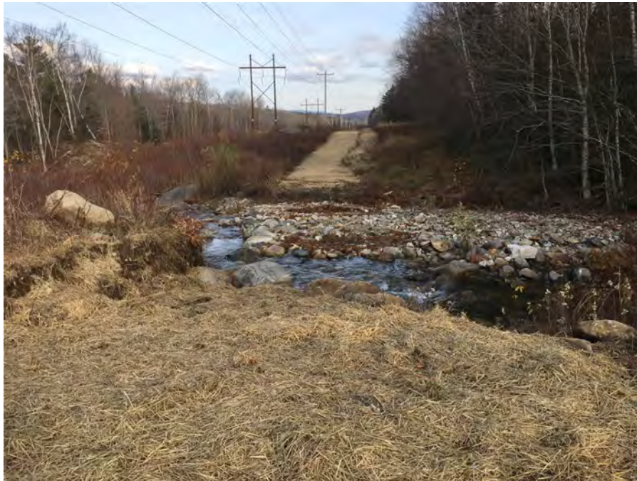
Photo 17. Existing ROW conditions near structure 212 at Cold Brook. Stantec, October 31, 2019.
