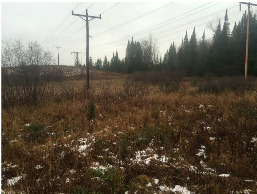
Photo 4. Existing ROW conditions near structure 29. Stantec, November 29, 2016.
