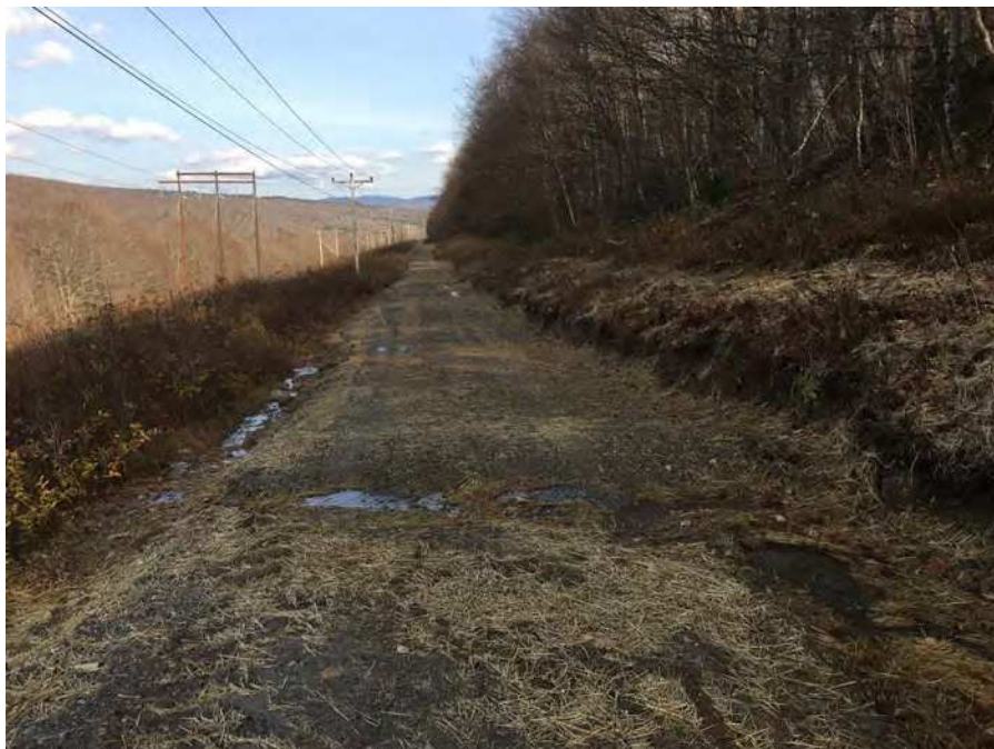
Photo 14. Existing ROW conditions near structure 200. Stantec, October 31, 2019.
