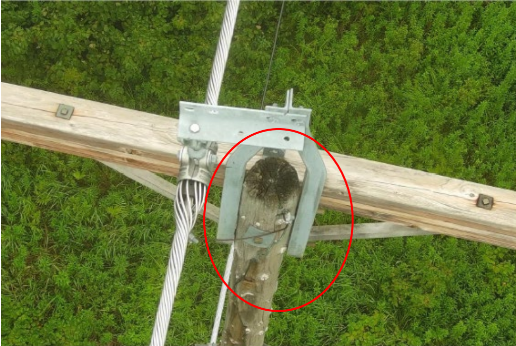
Line T198 Structure 119 Pole top rot, checking through crossarm attachment
