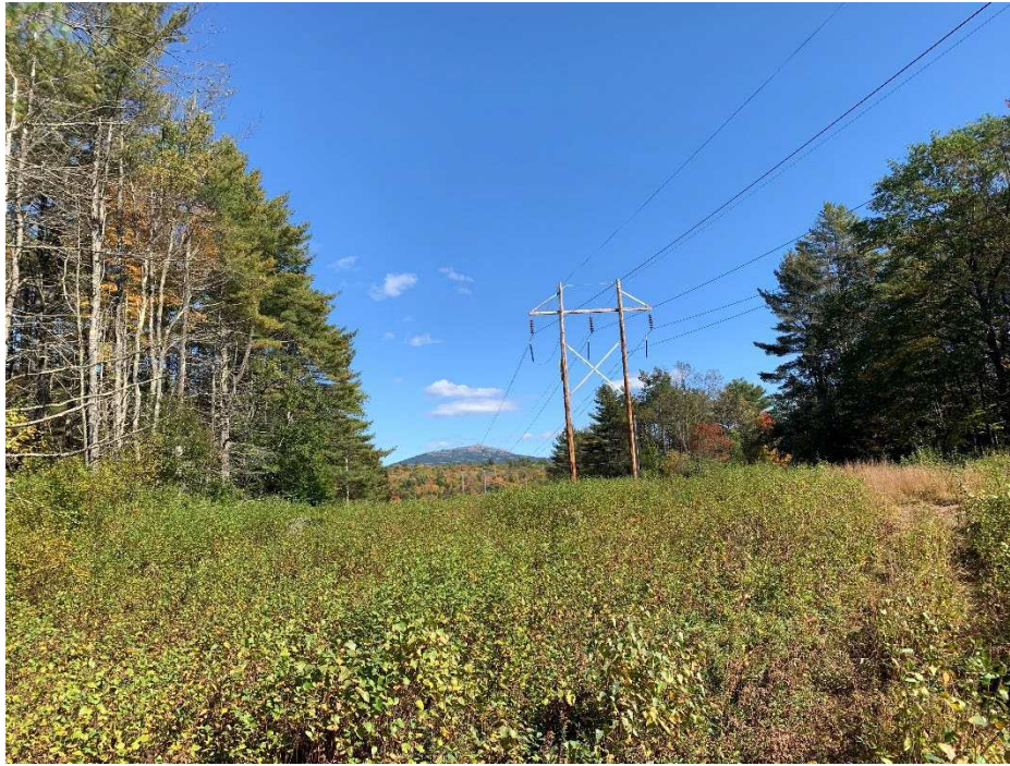
Photograph No. 5: Looking northwesterly at Structure 27.
