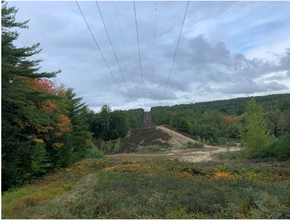
Photograph No. 5: Westerly view of Structure 70 from Structure 69.
