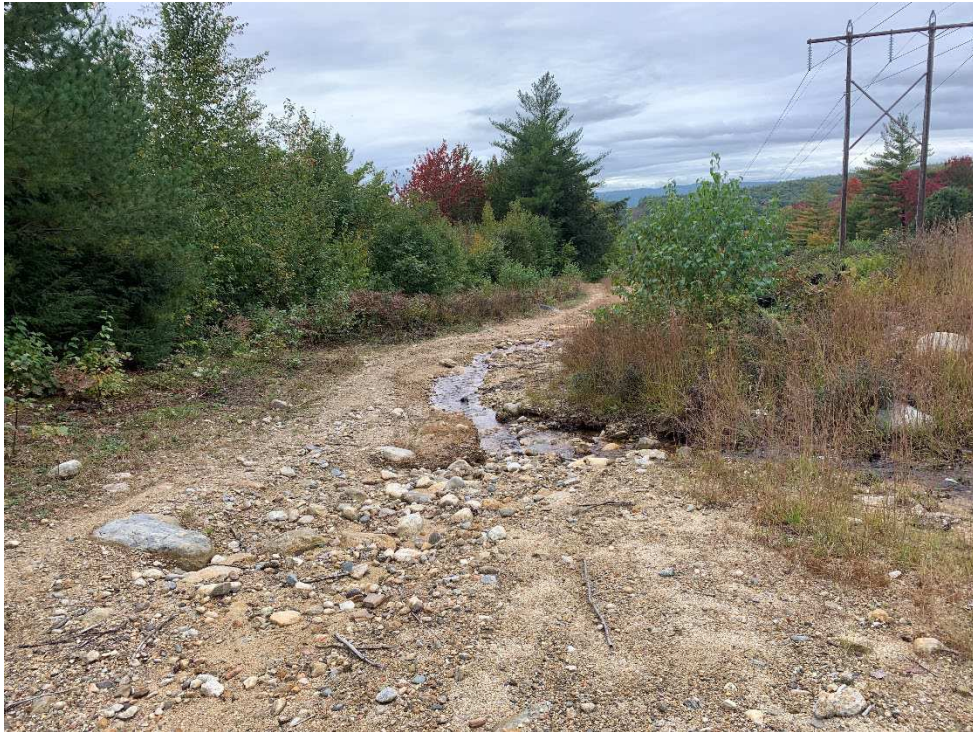
Photograph No. 9: Easterly view of proposed access towards Structure 63.
