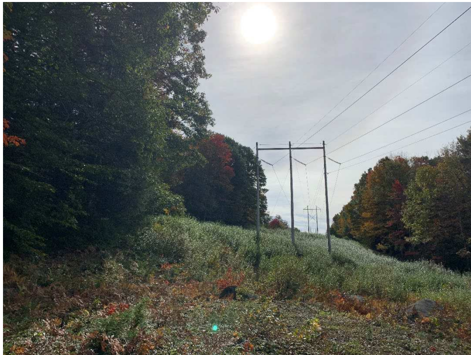
Photograph No. 22: Southerly view of Structure 10 (foreground) and Structure 9 (background).
