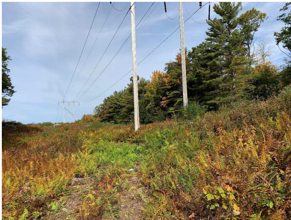
Photograph No. 20: Southeasterly view of Structure 13 (foreground) and Structure 12 (background).
