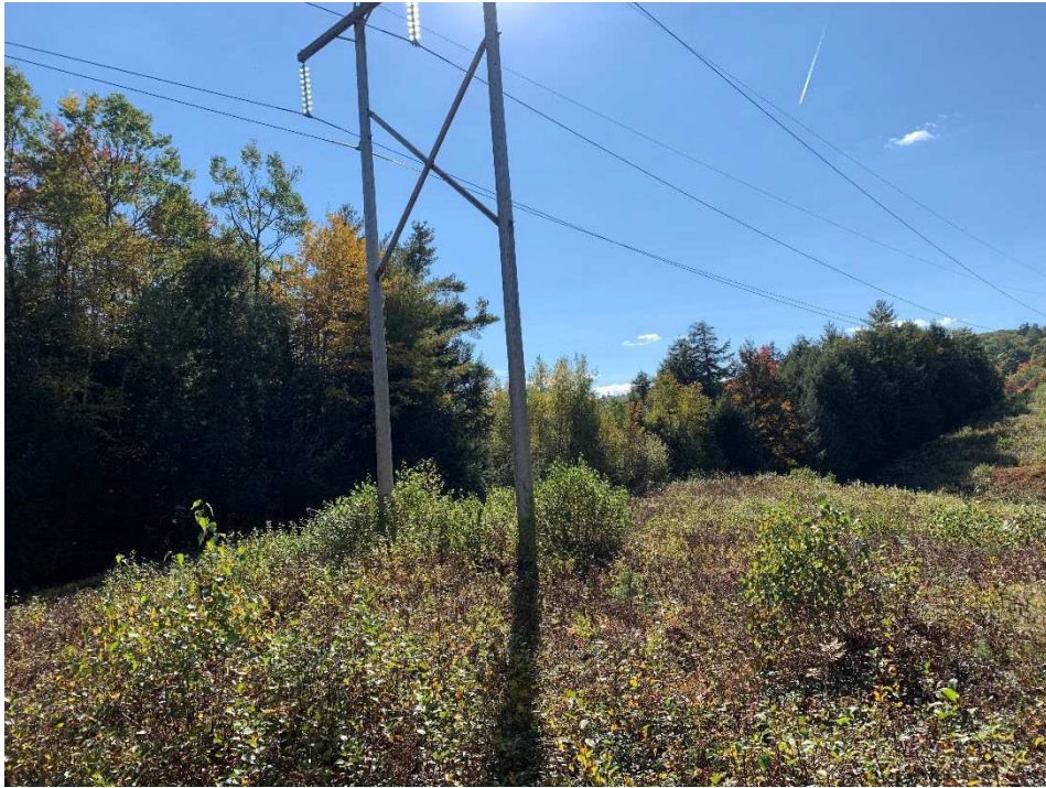
Photograph No. 3: Looking southerly at Structure 28 and proposed work pad area.
