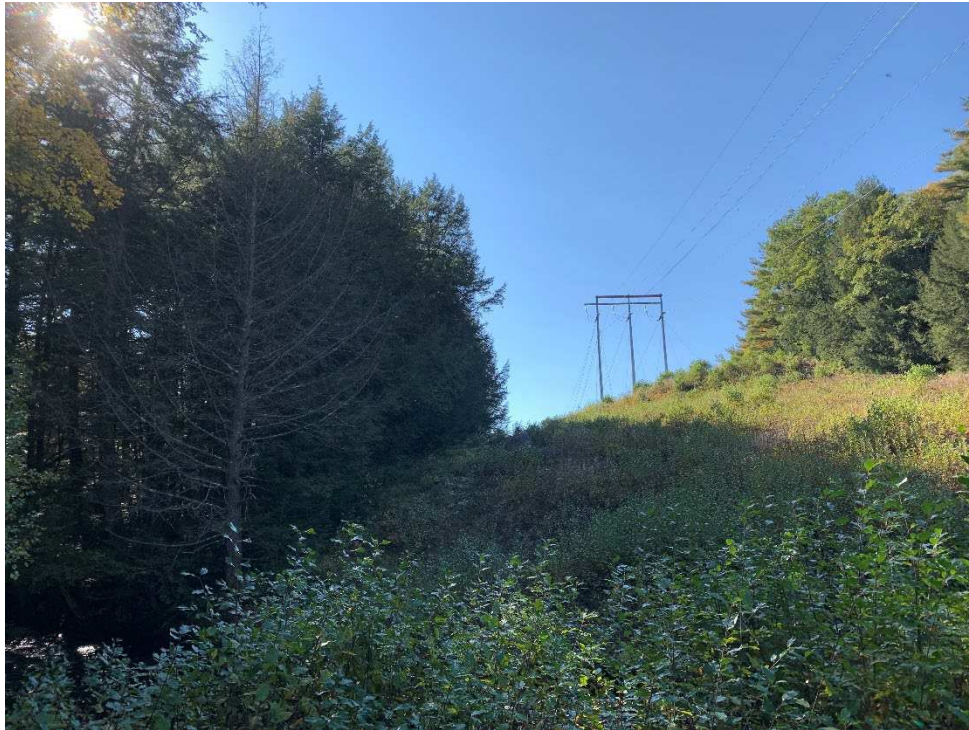
Photograph No. 1: Looking easterly from South Branch Ashuelot River toward Structure 29.
