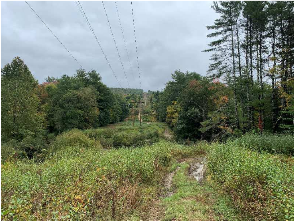
Photograph No. 1: Looking southeasterly from Structure 72 work area towards Structure 71.
