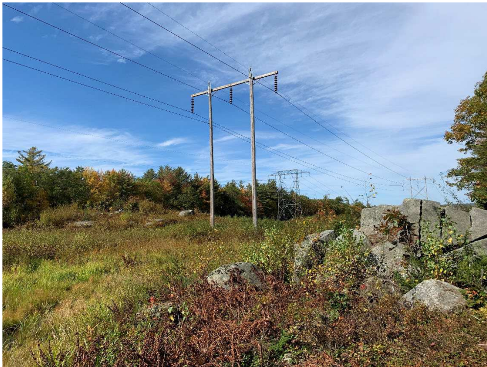
Photograph No. 16: Westerly view of Structure 17 and proposed work pad area.
