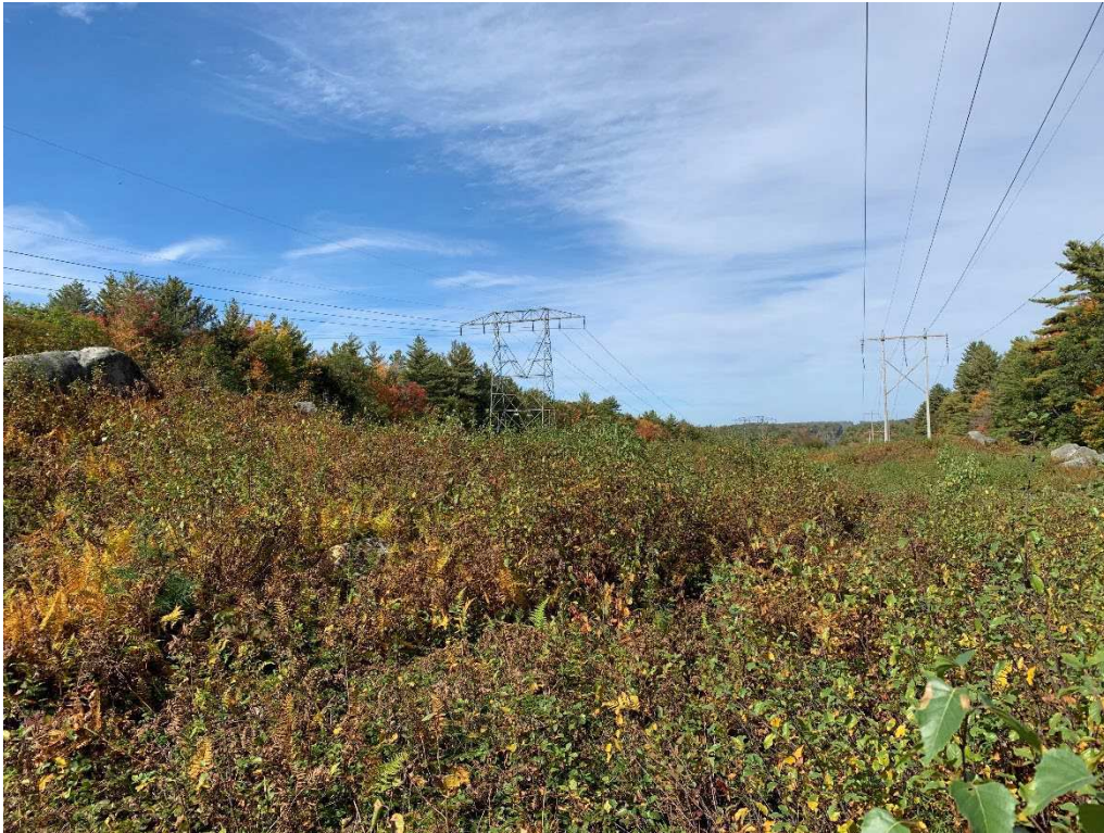
Photograph No. 15: Northwesterly view of Structure 19 from Structure 18.
