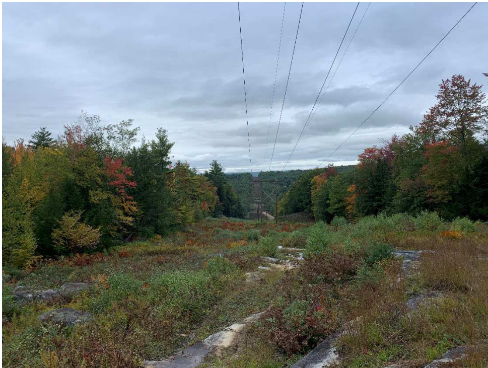
Photograph No. 8: Westerly view of Structure 66 from Structure 65.
