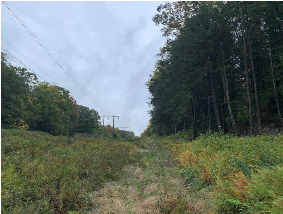
Photograph No. 6: Easterly view of proposed access to Structure 67 from Structure 68.
