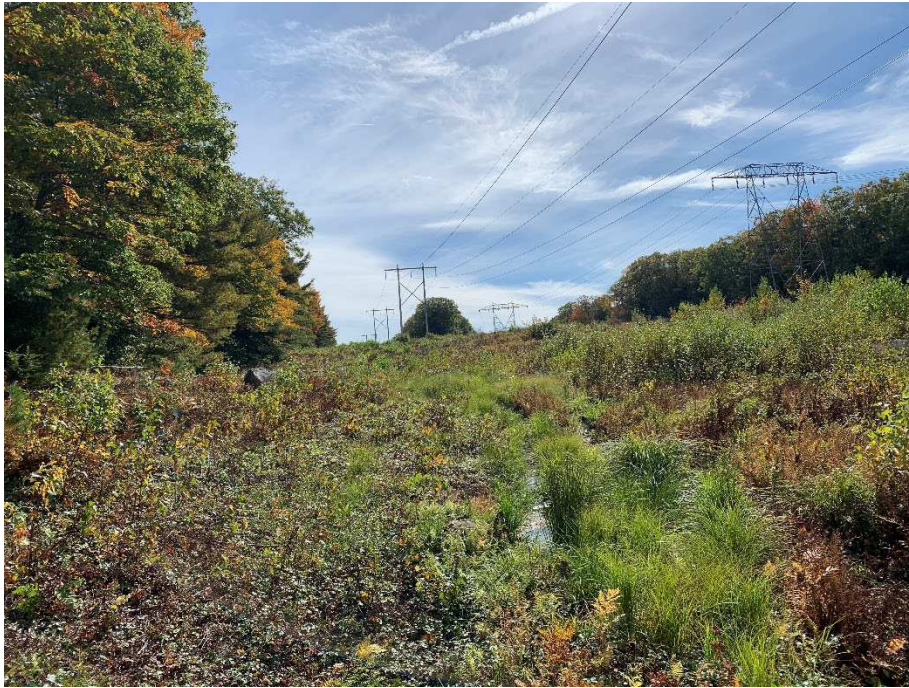
Photograph No. 17: Southeasterly view of proposed access to Structure 16 from Structure 17.
