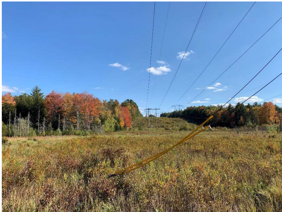
Photograph No. 12: Looking southeasterly toward Structure 22 from Structure 23.
