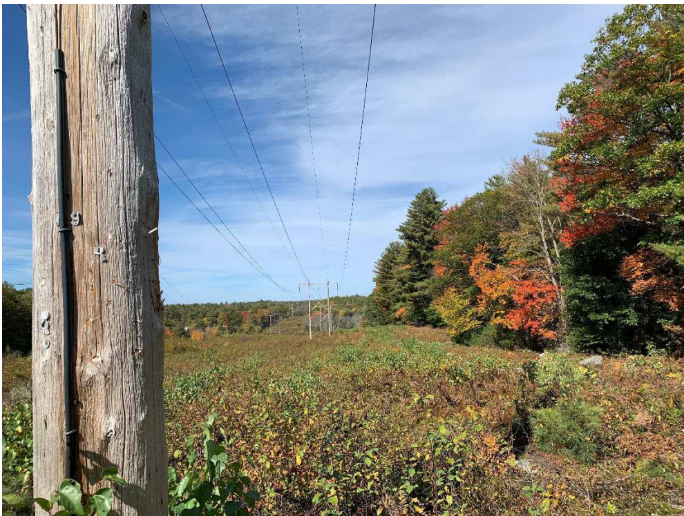
Photograph No. 14: Looking northwesterly at proposed access to Structures 20 and 21 from Structure 19.
