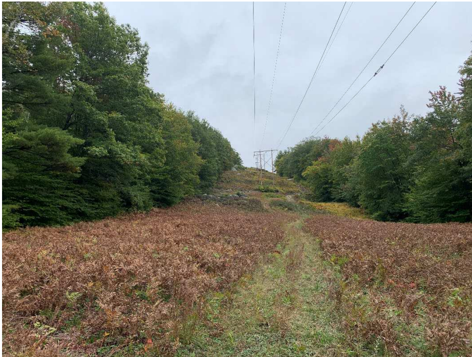
Photograph No. 12: Looking easterly at Structure 59 from Structure 60.
