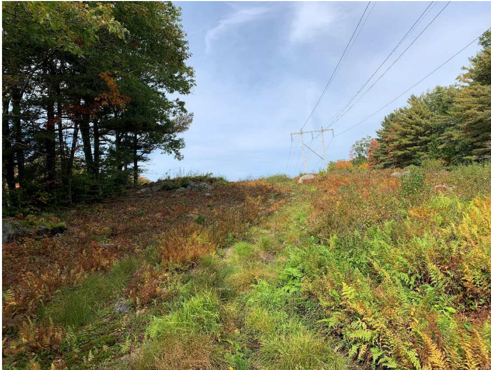
Photograph No. 19: Northerly view of proposed access to Structure 14 from Structure 13.
