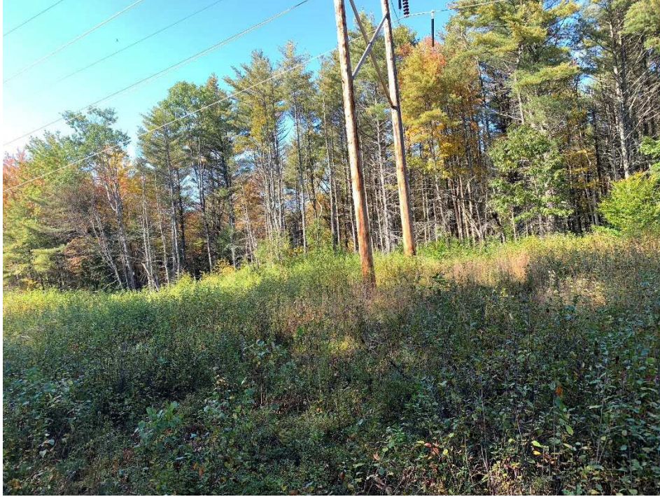
Photograph No. 7: Northerly view of Structure 26 and proposed work pad area.
