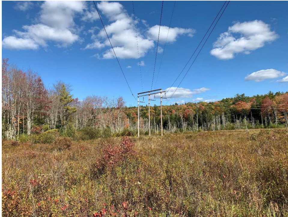
Photograph No. 11: Looking easterly at Structure 23.
