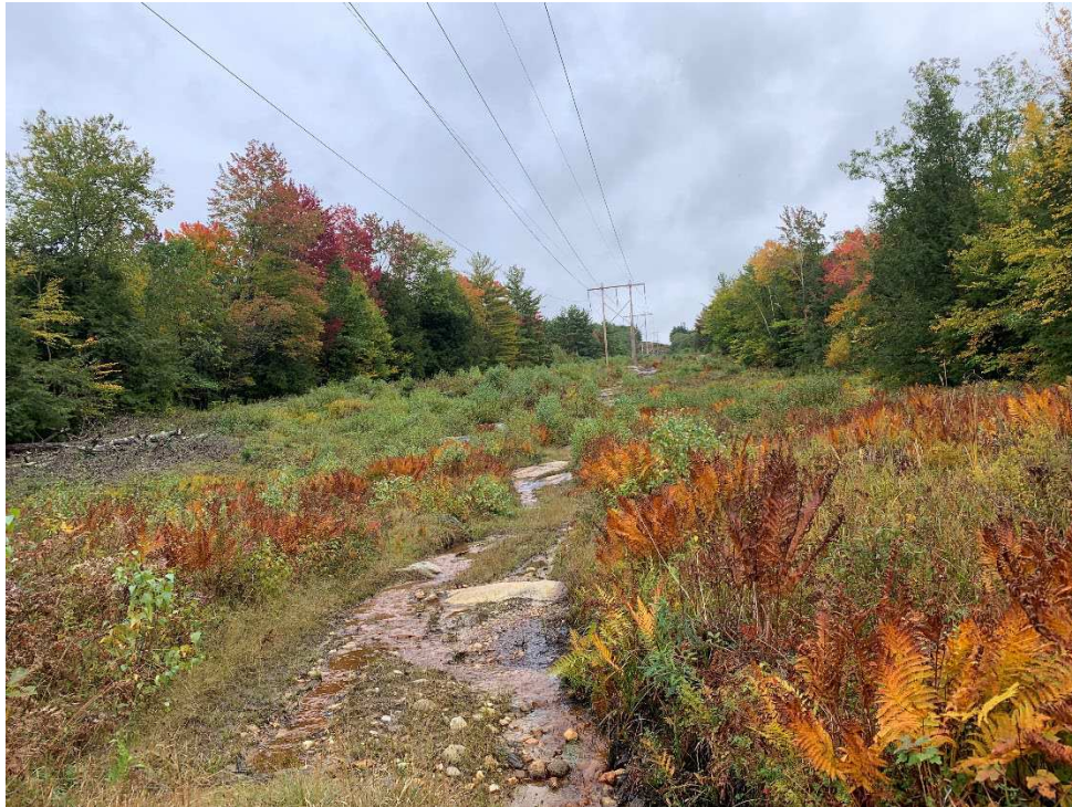
Photograph No. 7: Easterly view of Structure 65 from Structure 66. Timber matting to be utilized in this wetland.
