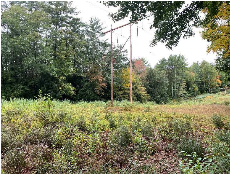
Photograph No. 2: Looking westerly at Structure 71 and proposed work pad area.
