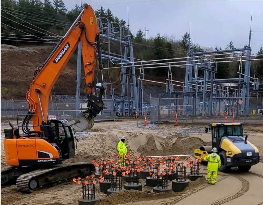
Drilled shafts installed
