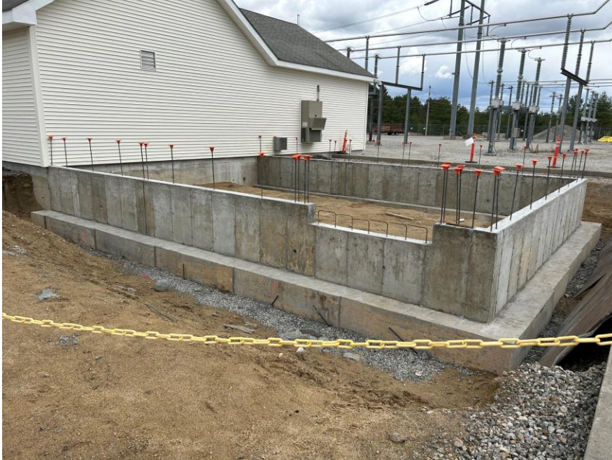
Left: Foundation for control house extension at Amherst
