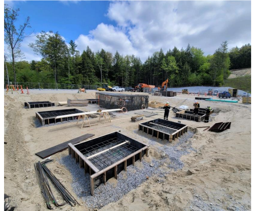
Foundation forms set up
