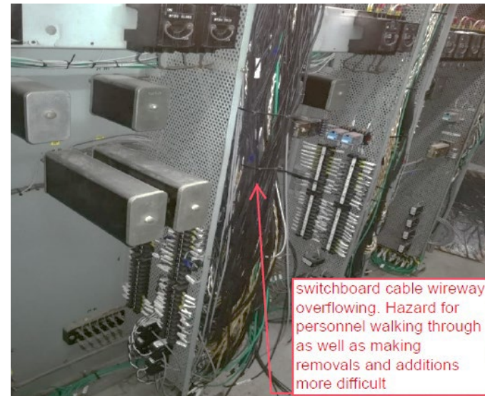
Overflowing switchboard
