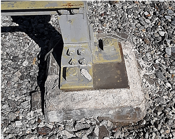
Foundation deterioration
