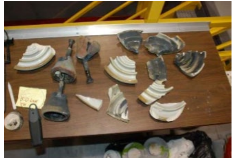
Fragments of Failed PINCO Insulator – Line 310
