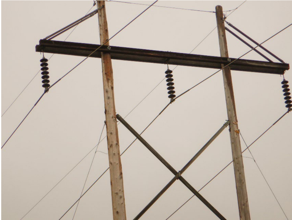
P145 - Structure 104 Example of existing H-frame structures
