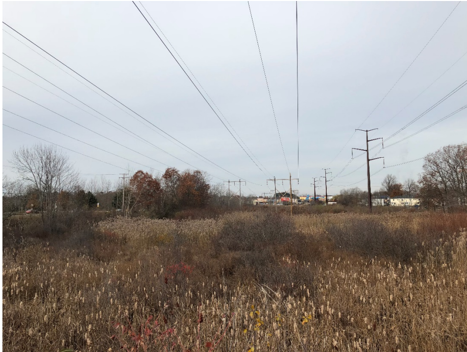
Photograph No. 9: View of the existing and maintained ROW corridor from within Wetland PW-27 facing north.
