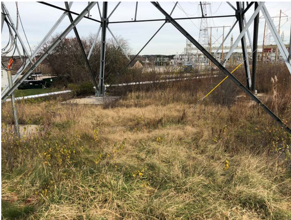
Photograph No. 14: View of the existing maintained ROW corridor from within Wetland PW-29. There are no proposed wetland impacts in this system
