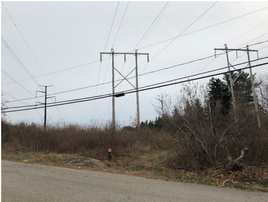
Photograph No. 2: View of U181 Structure 21 off Echo Avenue.
