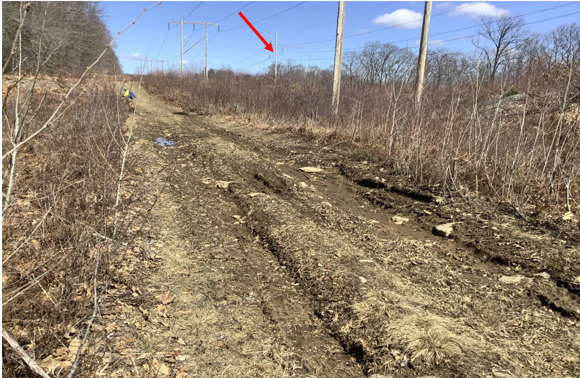
Photo 7: View north of the access road in the foreground and Structure 250 in the background (red arrow) in Franklin.
