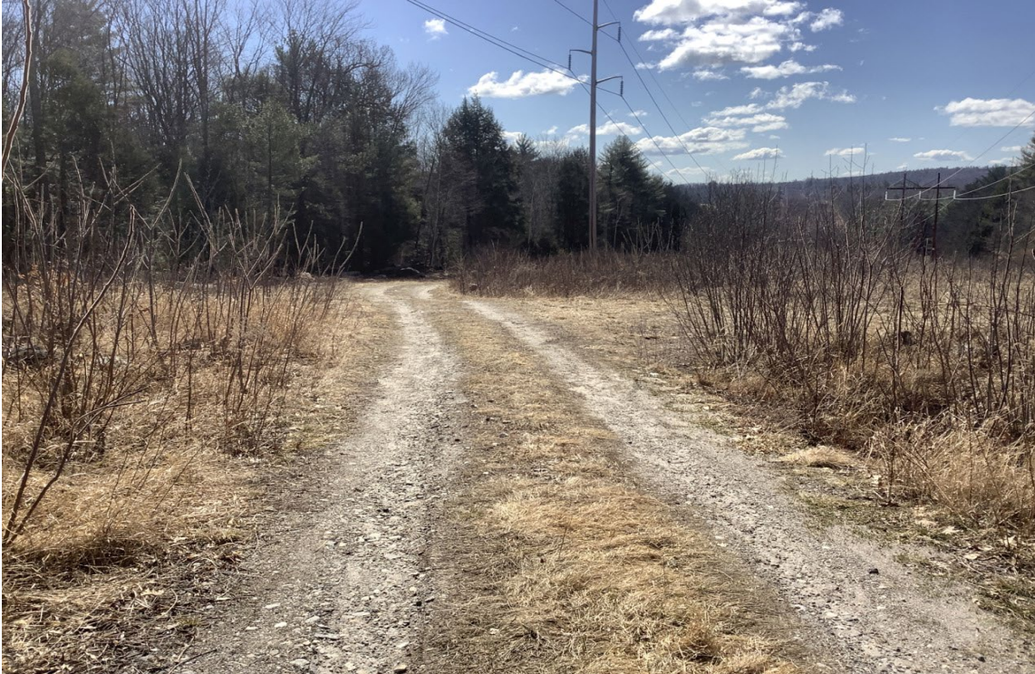
Photo 9: View southeast of Structure 246 with the existing access road in the foreground and proposed work pad area in the background in Franklin.
