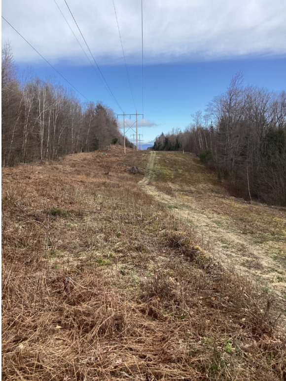
Photo 9. View north from near existing structure 77. Stantec, May 3, 2022.
