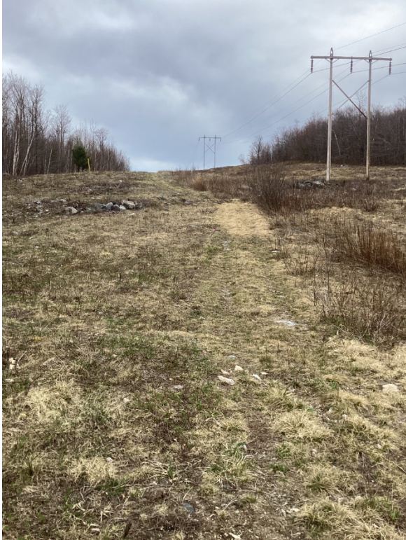
Photo 3. View east at steep slope leading up from near existing structure 8. Stantec, May 2, 2022.
