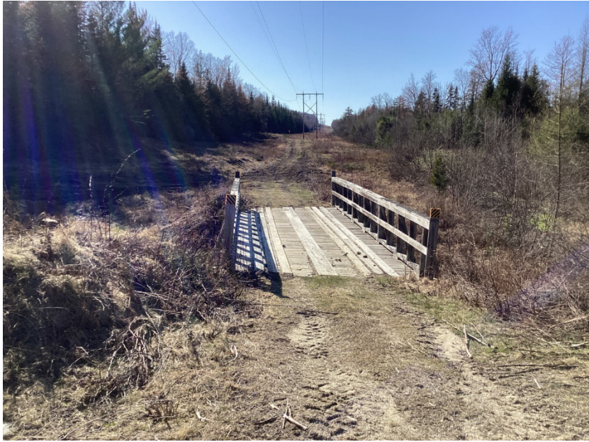
Photo 13. Existing snowmobile bridge, stream S50, near existing structure 135. Stantec, May 4, 2022.
