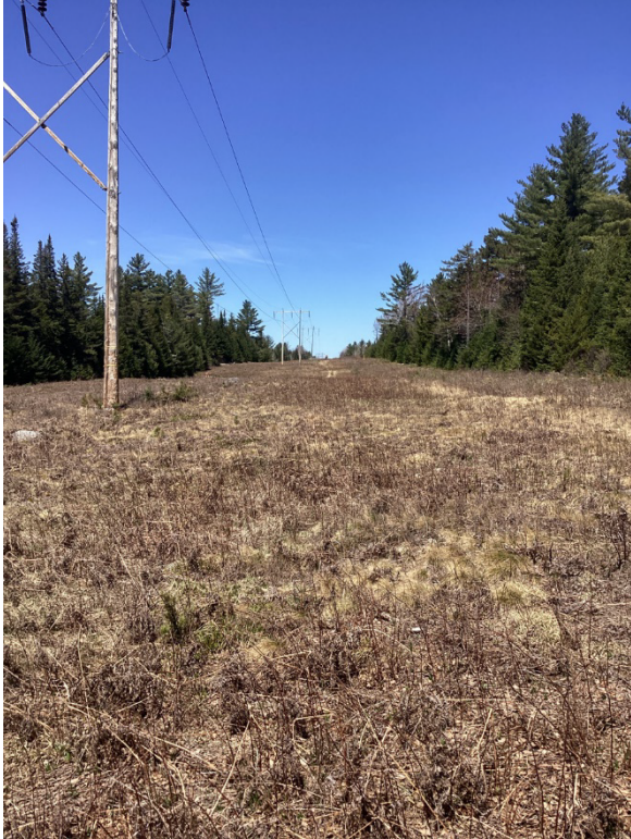
Photo 11. View north from near existing structure 102. Stantec, May 3, 2022.
