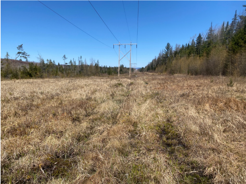
Photo 10. View north toward existing structure 95. Stantec, May 4, 2022.
