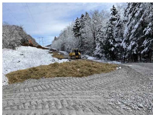
Gravel work pad area on the B112 Transmission Line in the WMNF with seedless mulch application
