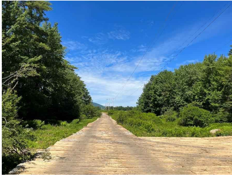
View of timber matting installed on the B112 Transmission Line (a similar project within the WMNF).
