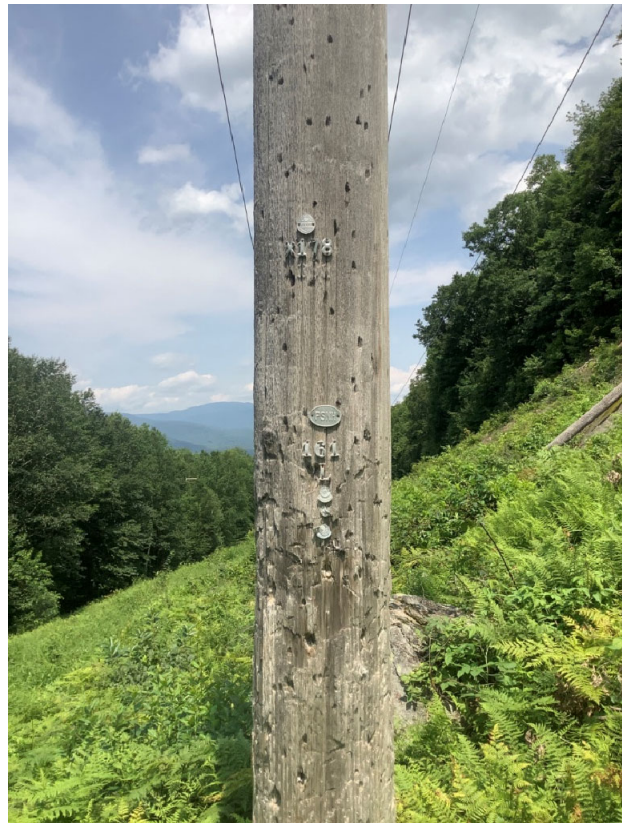
Photo 4: Closeup of Structure 161 with woodpecker and insect damage.
