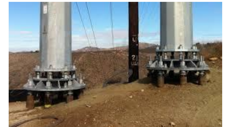
Micropile Transmission Structure Foundation
