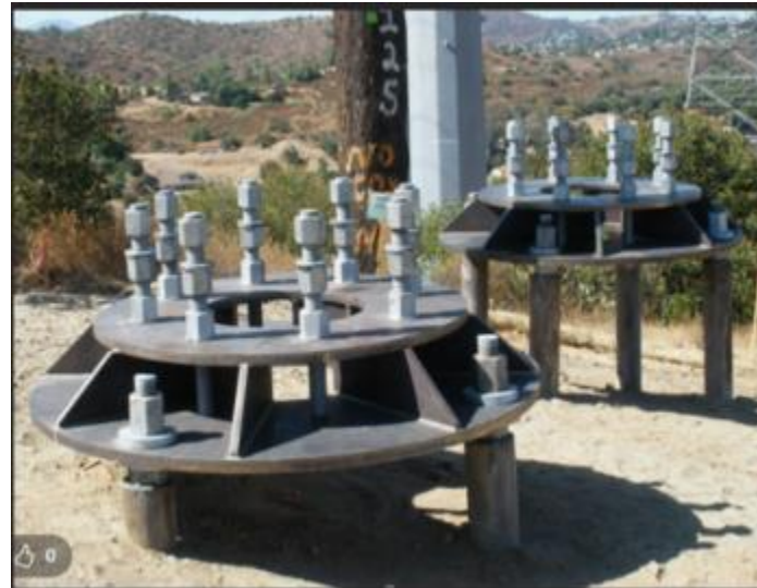
Micro Pile Foundations - Helicopter
