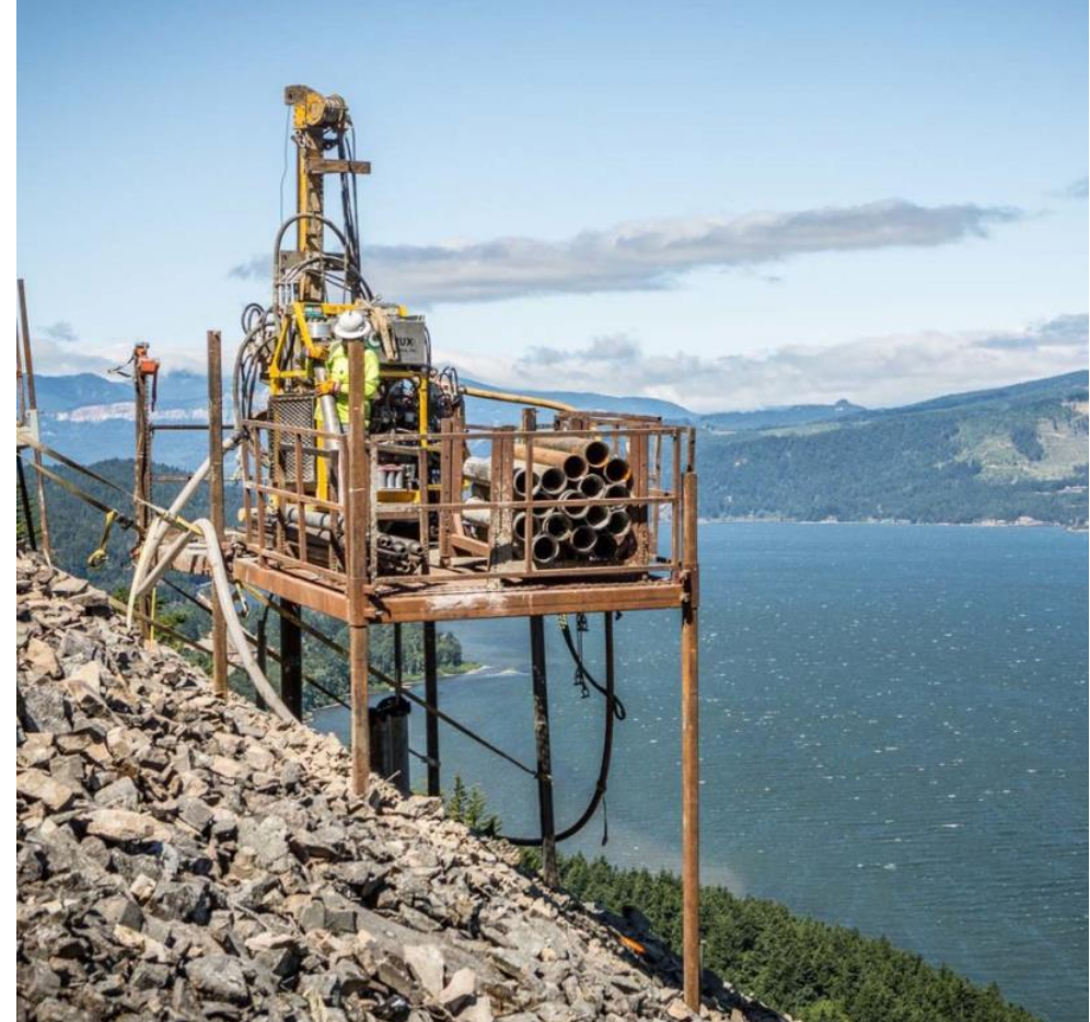
Drilling platform for micropiles
