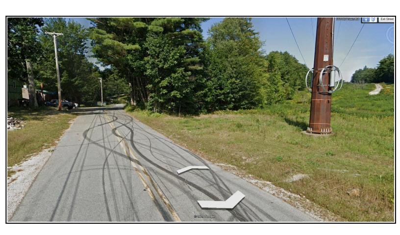
Above, A-111 monopole with splice "boxes" for the Optical Ground Wire.
