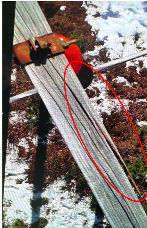
Cracked Cross Arm
