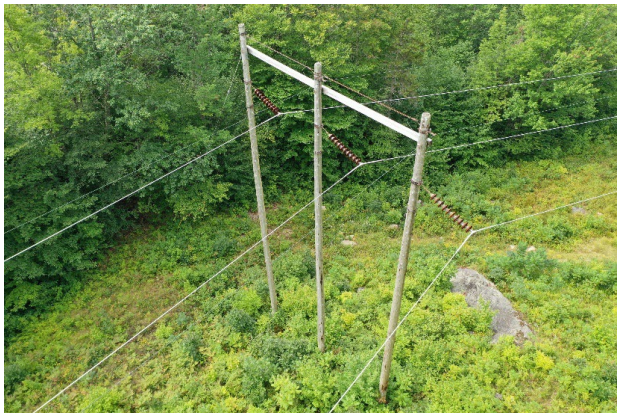
Examples of existing structures to be removed
