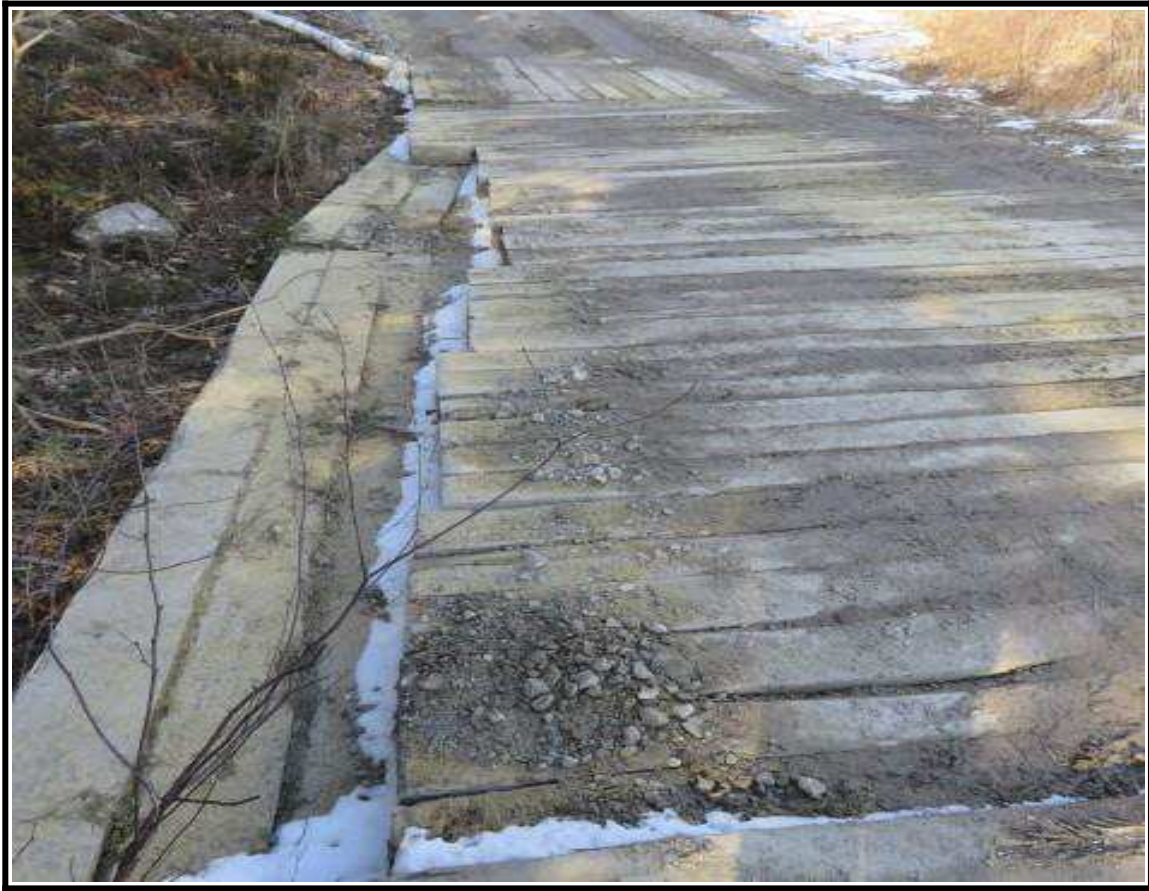
(Right: U-181/E-194 12/2/2024) Silty gravel dump above wetland.
