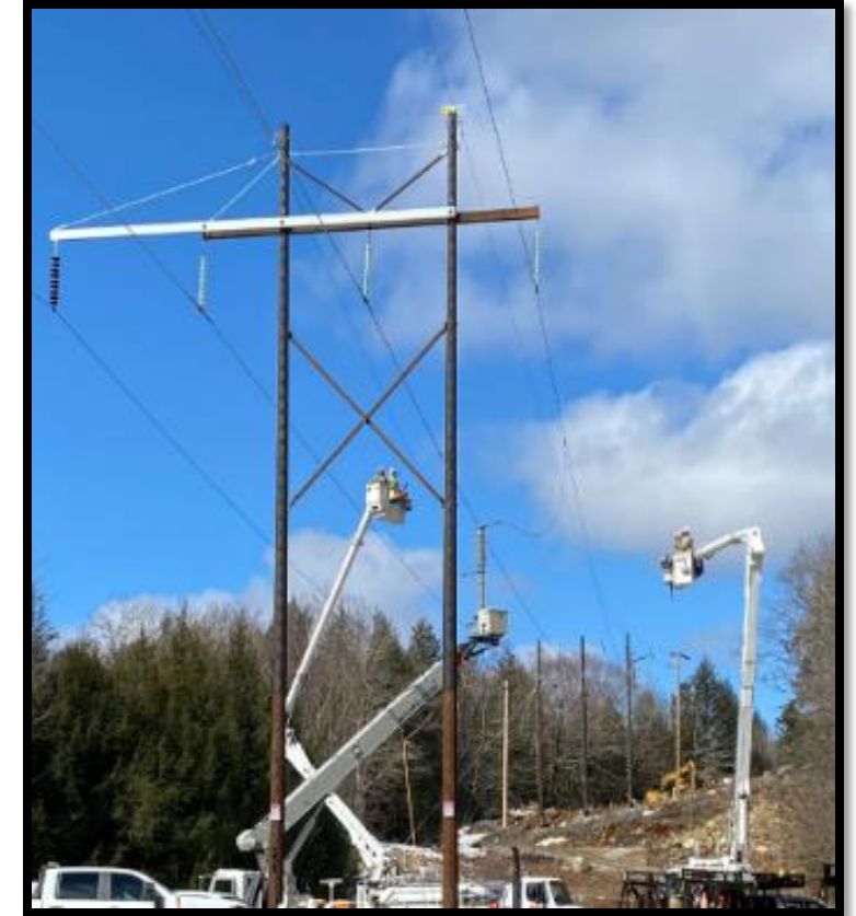
Typical live-line conductor replacement
