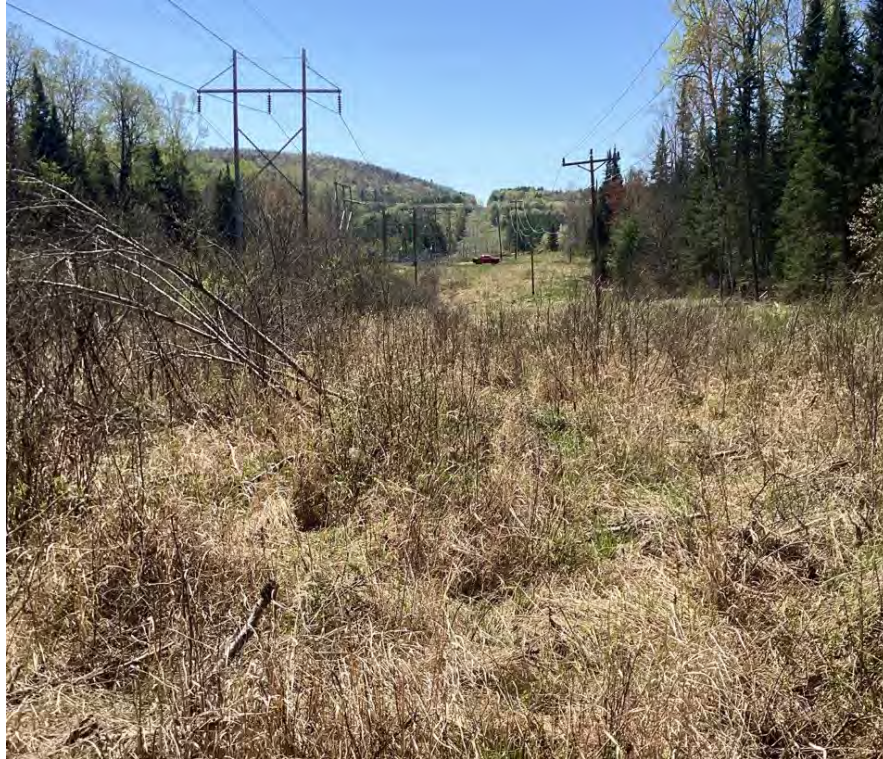
Photo 1. Shrub-dominated ROW uplands looking northeast to structure 405. May 8, 2023.
