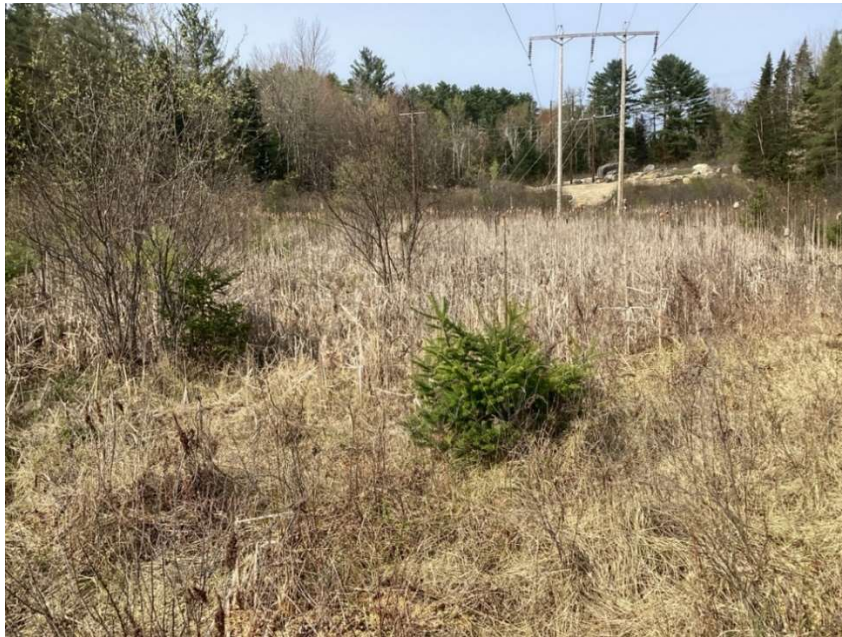
Photo 3. Wetland W018. View northeast towards proposed structure 426. May 2023.
