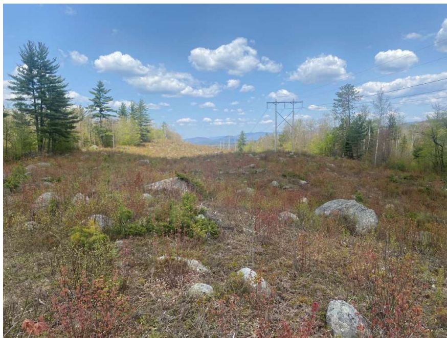
Photo 18. Representative ROW upland north of proposed structure 520. May 2023.
