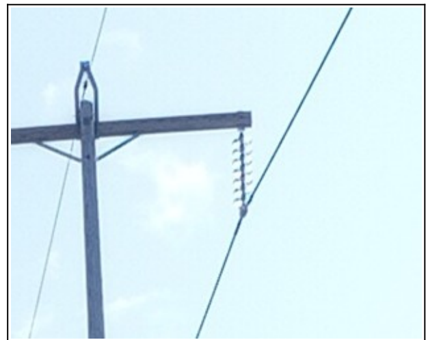
Right: X-178 line, not rebuilt, 795 ASCR conductor, 7 insulators. Insulators and
