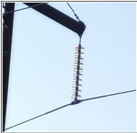
Left: rebuilt S-136 line 795 ASCR conductor 10 insulators
