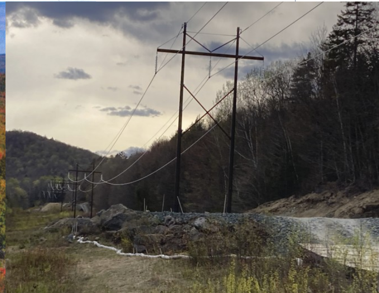
O-154 after rebuild
