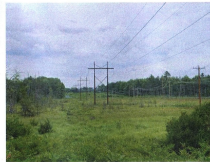
D142 Construction Complete 2022
