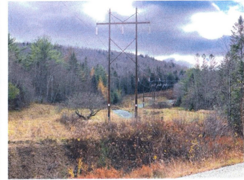
O154 Restoration –Construction Complete 2023
