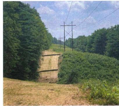
E115 Restoration –Construction Complete 2023
