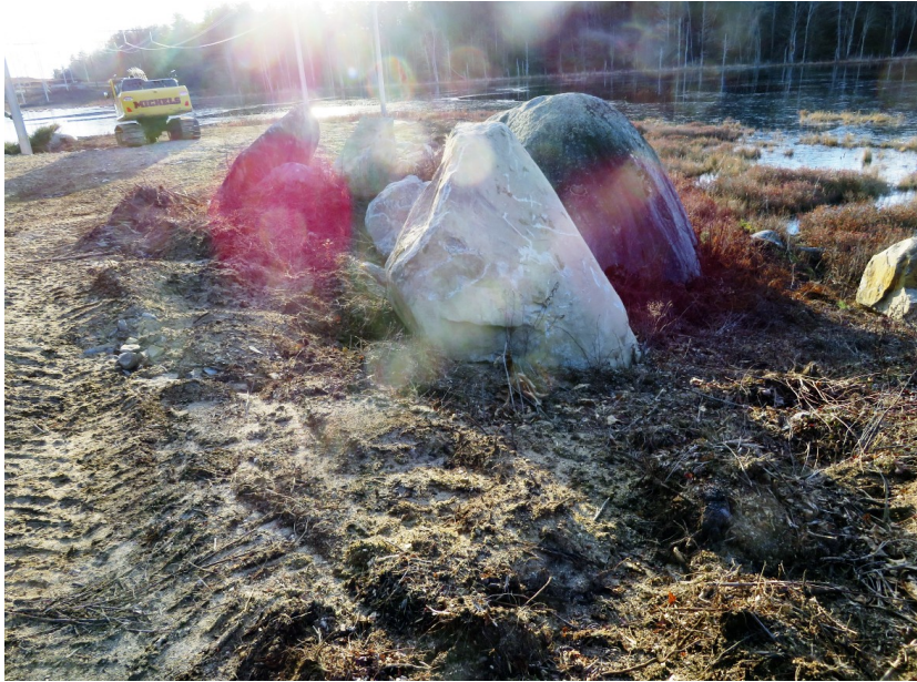
Eversource construction close up; another “Asset Condition” project.
