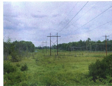
D142 Construction Complete 2022
