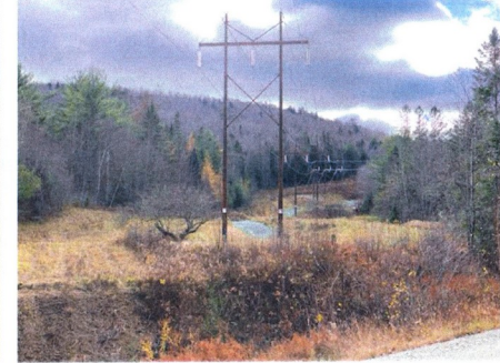
O154 Restoration –Construction Complete 2023
