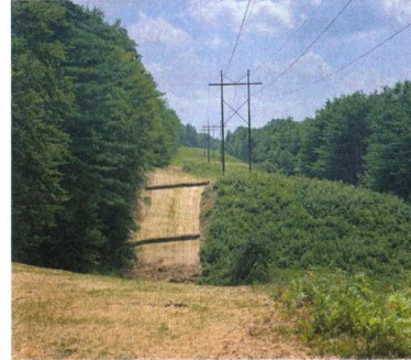
E115 Restoration –Construction Complete 2023
