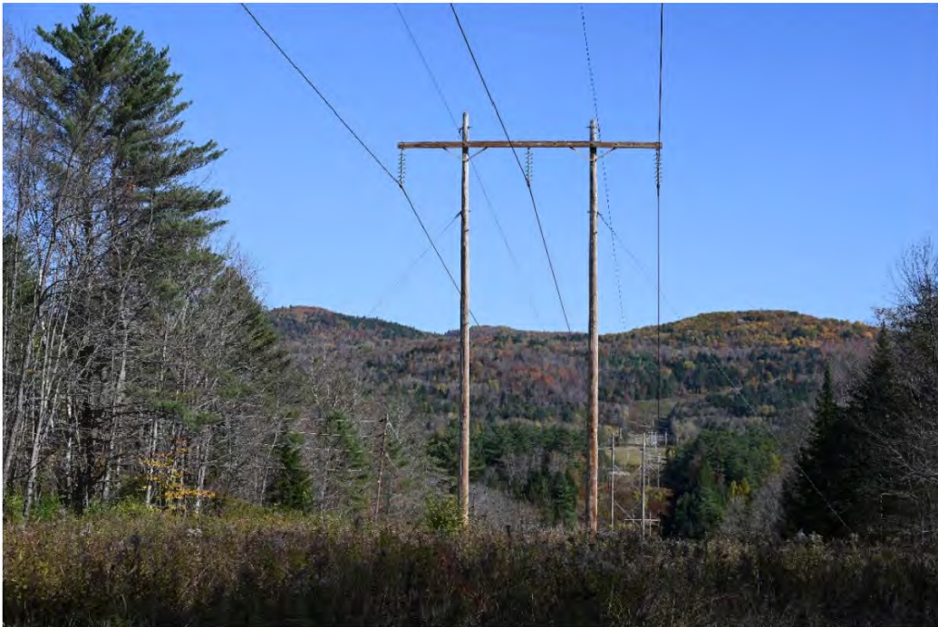
Photo A1: wood H-Frame structure #394, 48.3 ft tall, viewing distance 125 ft (50mm focal length)
