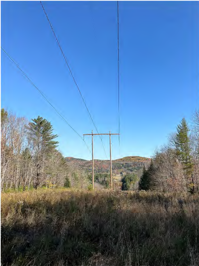
Photo A3: wood H-Frame structure #394, 48.3 ft tall, viewing distance 140 ft (24mm focal length)
