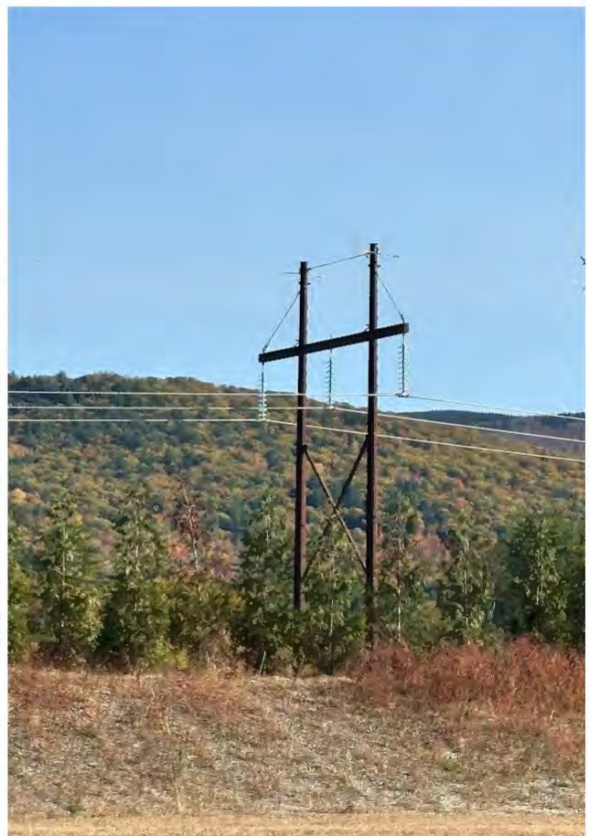
Photo B4: weathering steel H-Frame structure #41, 51.0 ft tall, viewing distance 325 ft
