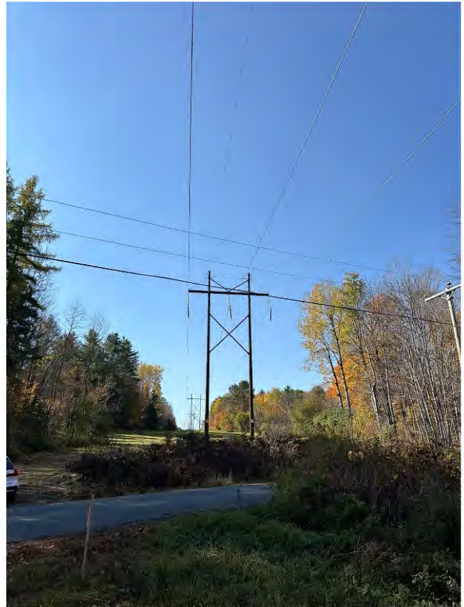
Photo A2: weathering steel H-Frame structure #393, 65.5 ft tall, viewing distance 140 ft (24mm focal length)
