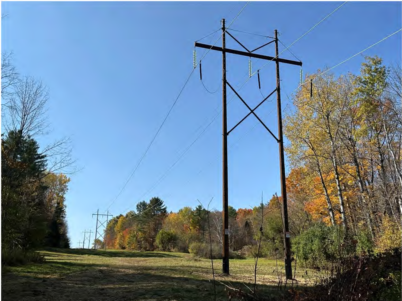
Photo A5: weathering steel H-Frame structure #393, height of 65.5 ft, viewing distance of 90 ft / wood H-Frame structures #389 to 392, height range 45.8 to 58.2 ft, viewing distance of 700 ft to 2,300 ft (37mm focal length)
