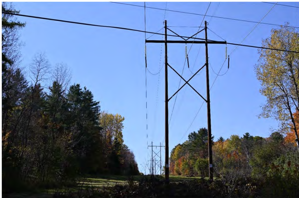
Photo A2: weathering steel H-Frame structure #393, 65.5 ft tall, viewing distance 155 ft (50mm focal length)
