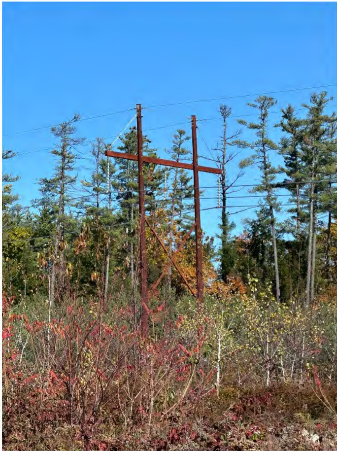
Photo B3: weathering steel H-Frame structure #42, 50.2 ft tall, viewing distance 265 ft
