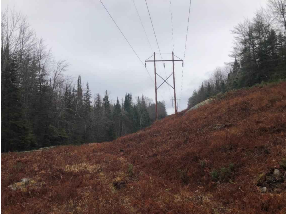
Photograph No. 83: Looking northeasterly at proposed access toward Structure 377.
