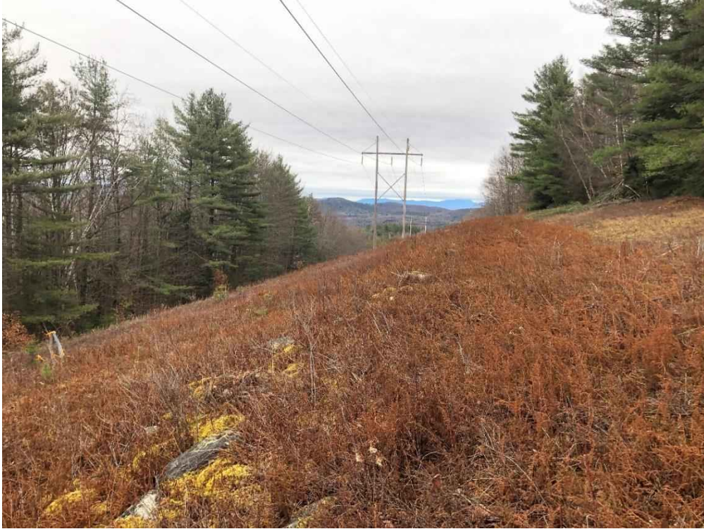
Photograph No. 91: Looking northwesterly at proposed access toward Structure 385.
