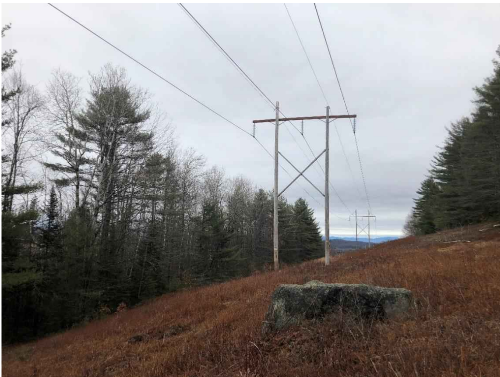
Photograph No. 90: Looking northeasterly at proposed access toward Structure 384.
