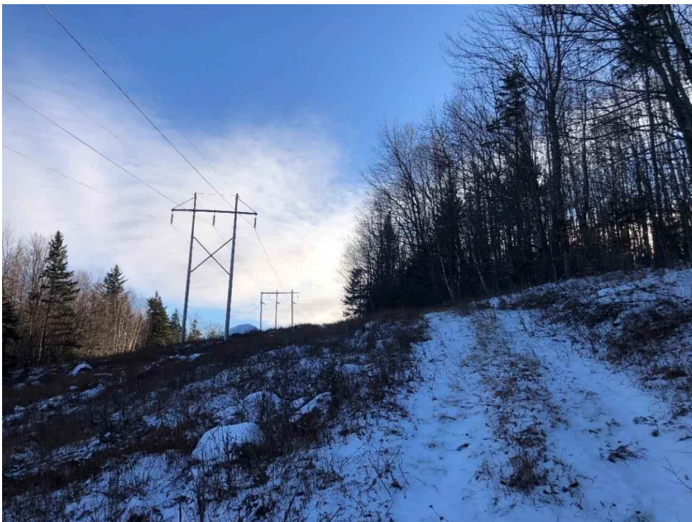
Photograph No. 32: Looking southerly at proposed access toward Structure 326.
