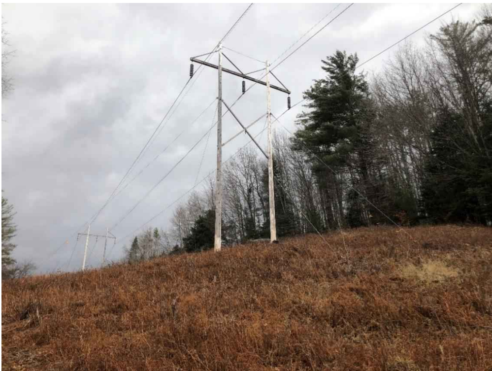
Photograph No. 76: Looking northerly at proposed access and work pad location for Structure 371.
