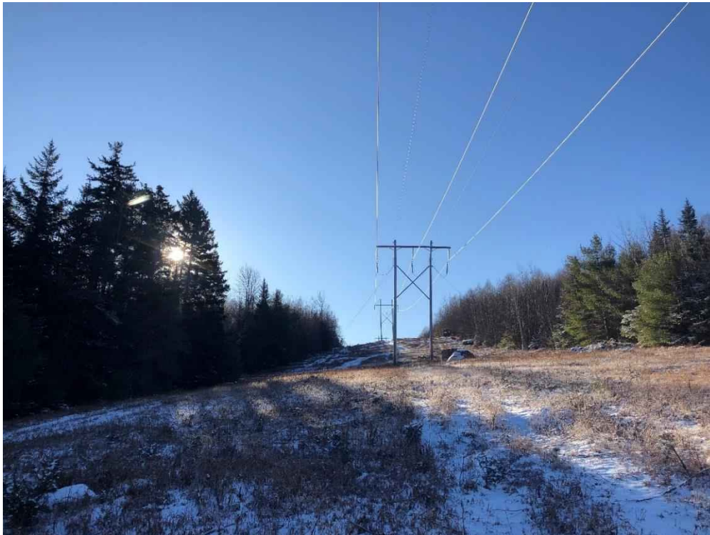
Photograph No. 44: Looking southerly at proposed access toward Structure 338.
