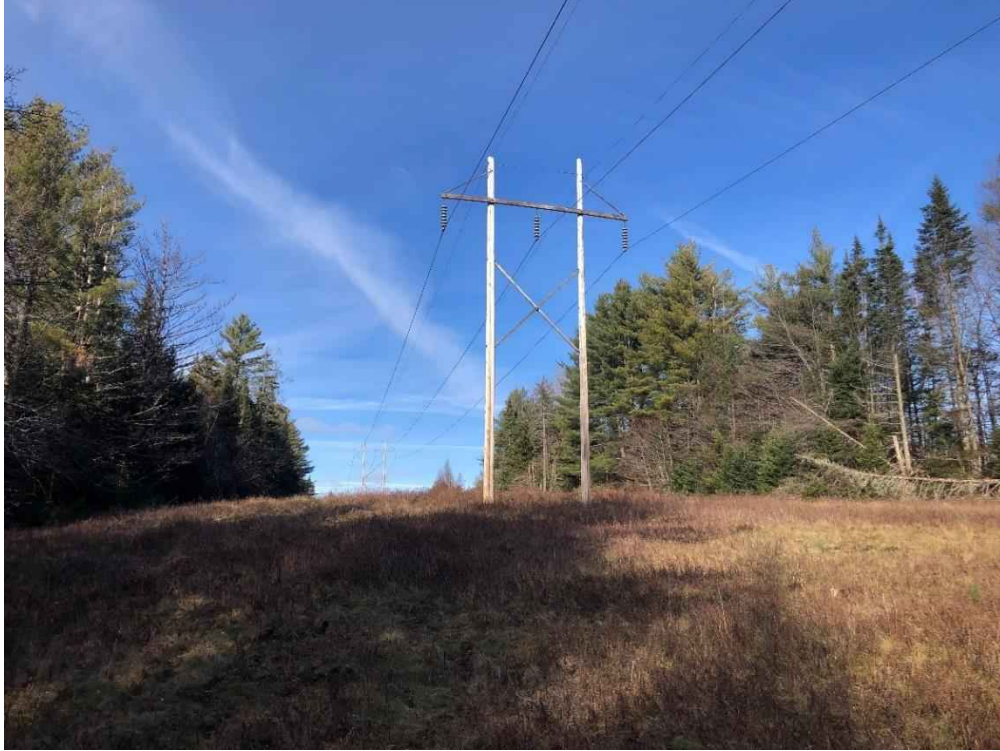
Photograph No. 61: Looking at proposed access and work pad location for Structure 356.
