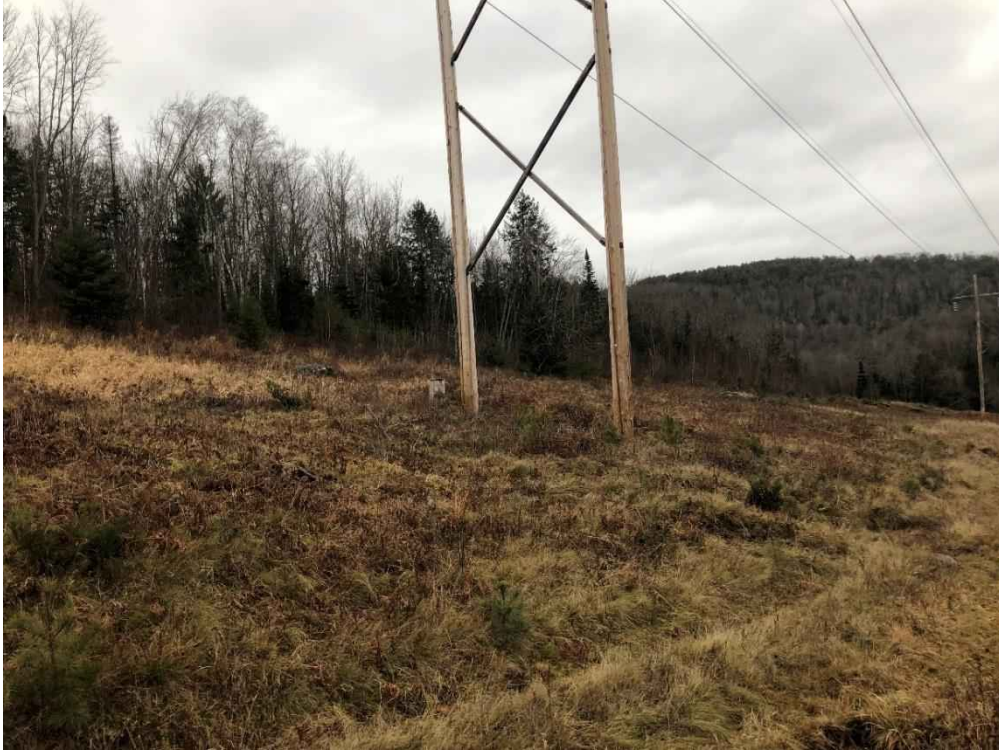
Photograph No. 73: Looking northwesterly at proposed work pad location for Structure 368.
