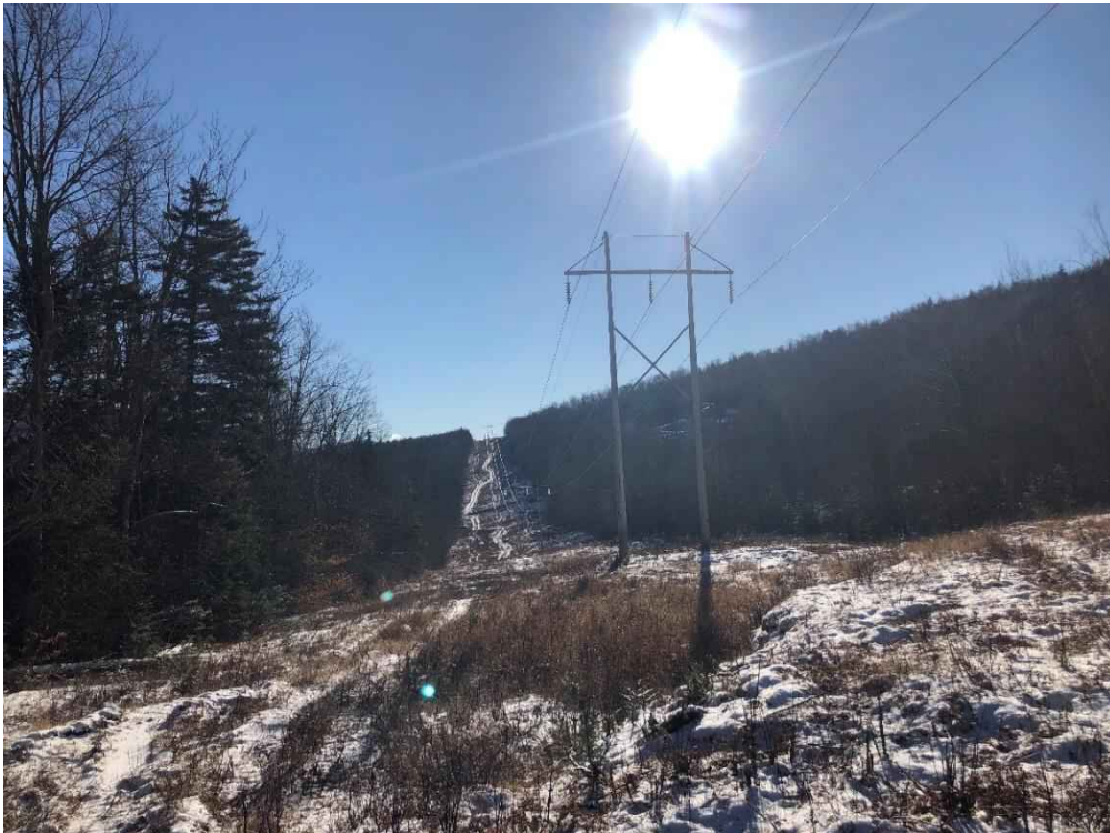
Photograph No. 38: Looking southerly at proposed access toward Structure 332.
