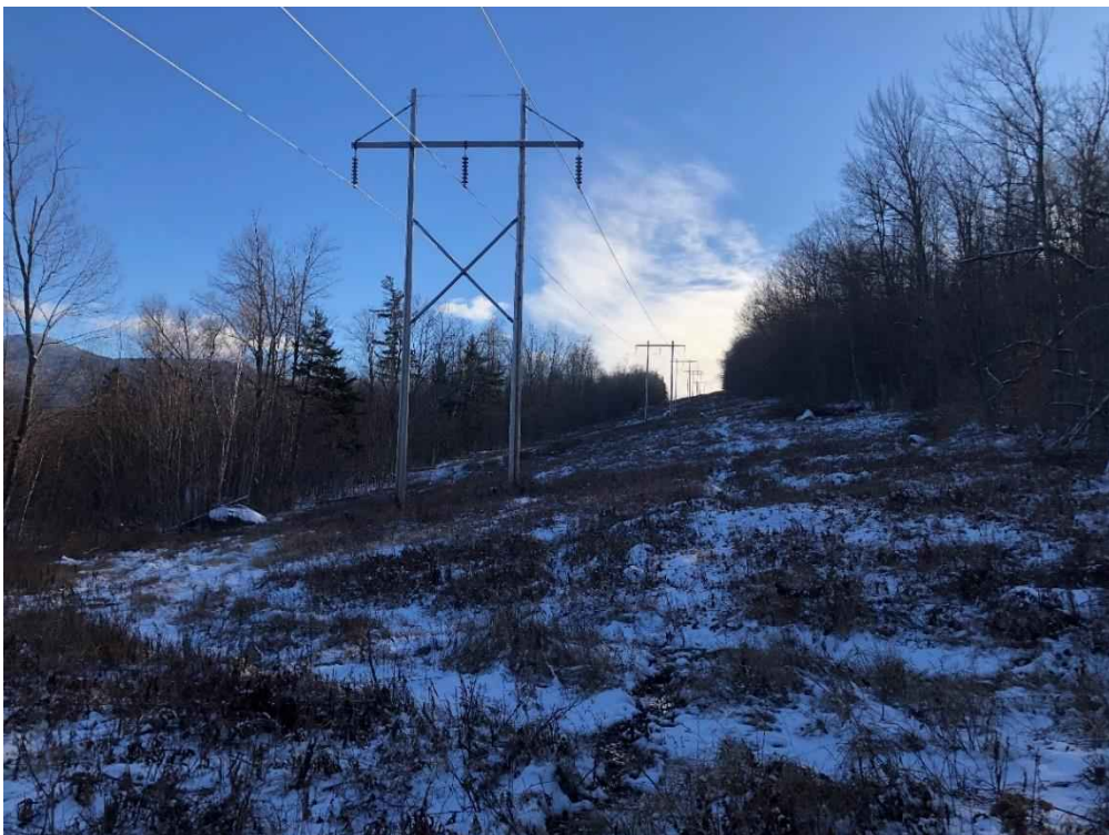
Photograph No. 36: Looking southerly at proposed access toward Structure 330.
