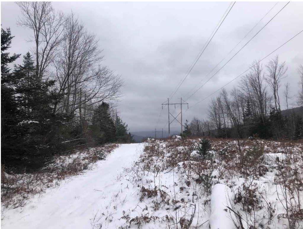
Photograph No. 22: Looking southerly at proposed access toward Structure 316.
