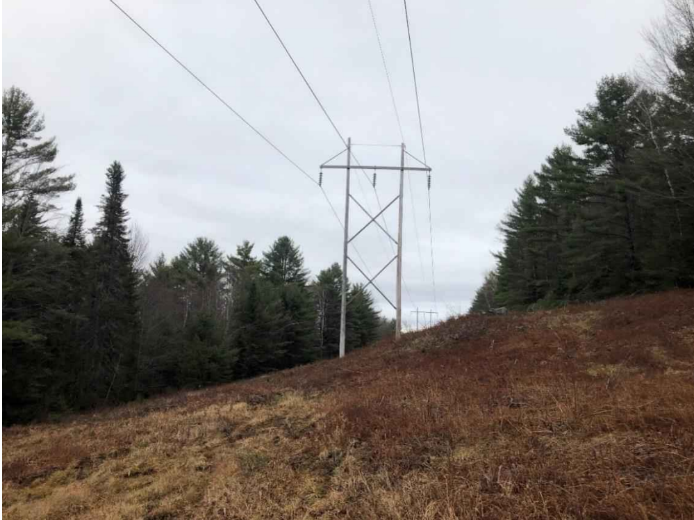
Photograph No. 89: Looking northeasterly at proposed access toward Structure 383.
