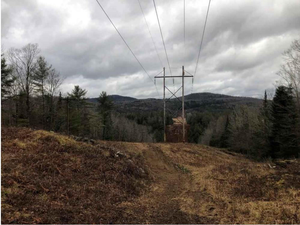
Photograph No. 101: Looking northeasterly at proposed access toward Structure 395.
