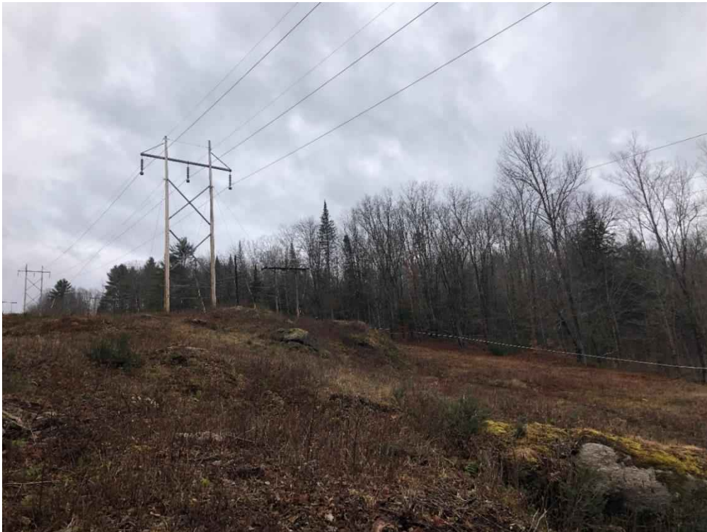
Photograph No. 102: Looking southwesterly at proposed access toward Structure 396.
