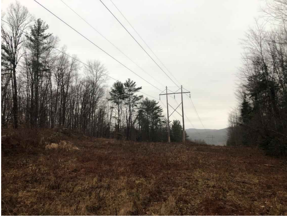
Photograph No. 97: Looking northeasterly at proposed access toward Structure 391.
