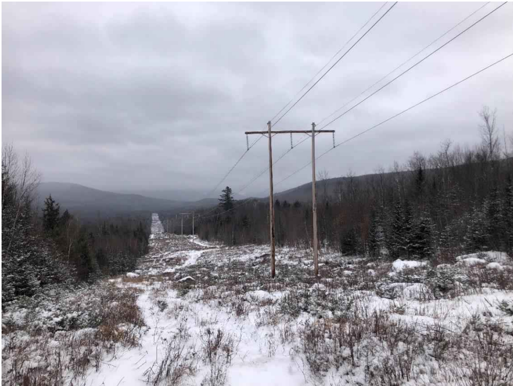
Photograph No. 26: Looking southerly at proposed access toward Structure 320.
