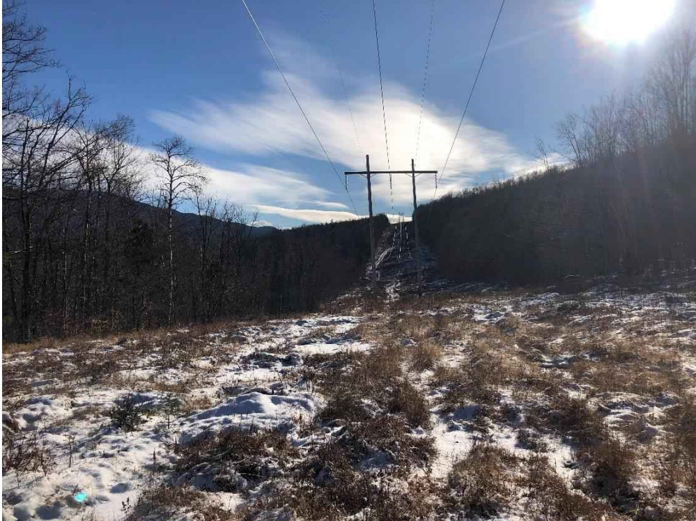
Photograph No. 37: Looking southerly at proposed access toward Structure 331.
