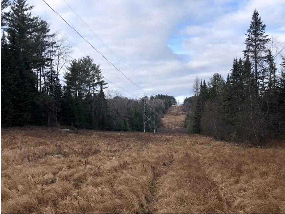
Photograph No. 65: looking northerly at proposed access toward Structure 360.
