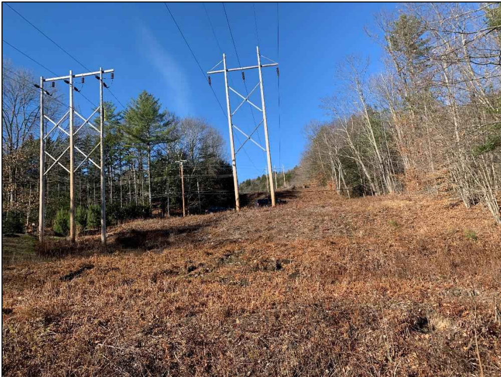
Photograph No. 6: Looking westerly at proposed access toward Structure 175 (right).
