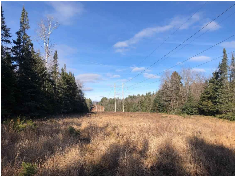
Photograph No. 58: Looking northerly at proposed access toward Structure 353.
