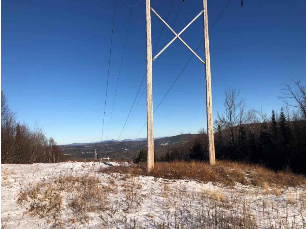
Photograph No. 43: Looking southerly at proposed work pad location for Structure 337.
