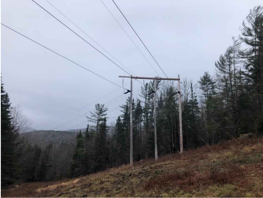
Photograph No. 79: Looking southwesterly at proposed access toward Structure 374.
