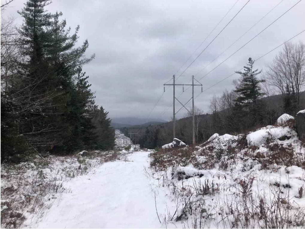
Photograph No. 21: Looking southerly at proposed access toward Structure 315.
