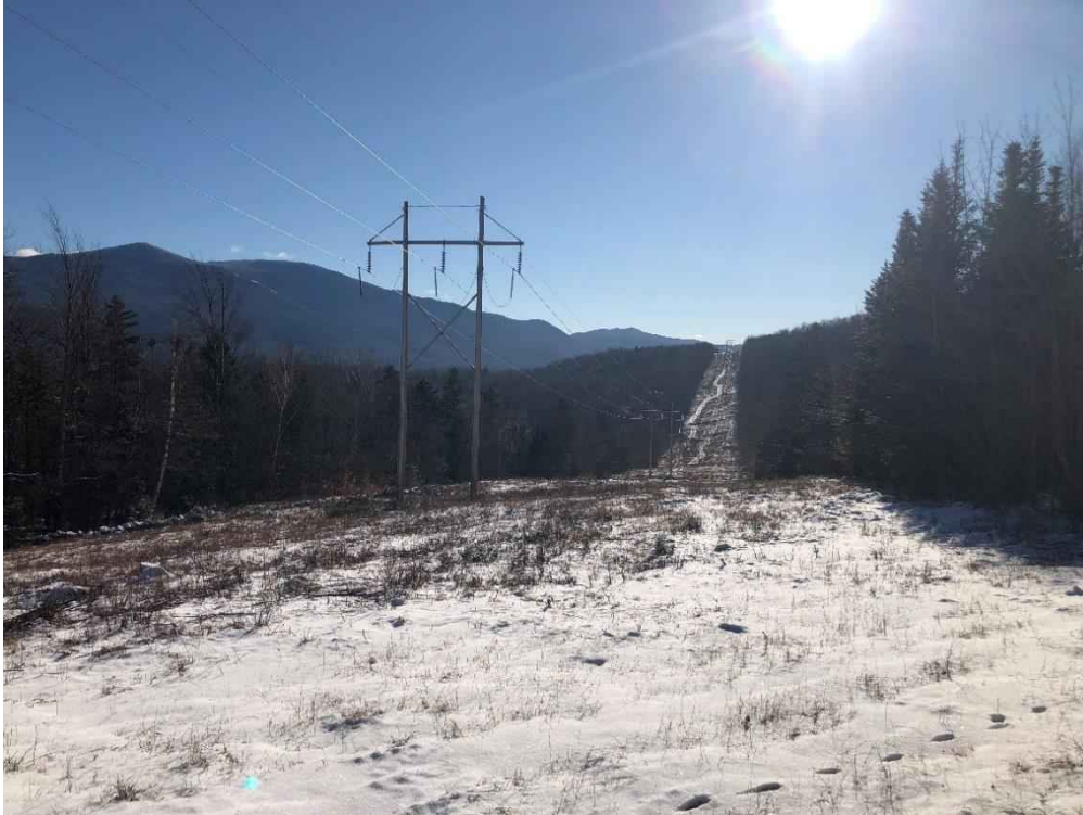
Photograph No. 39: Looking southerly at proposed access toward Structure 333.
