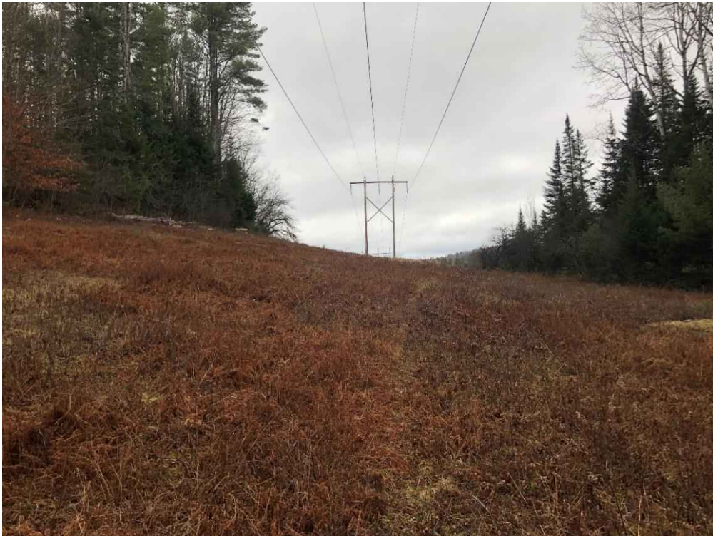
Photograph No. 72: Looking northerly at proposed access toward Structure 367.
