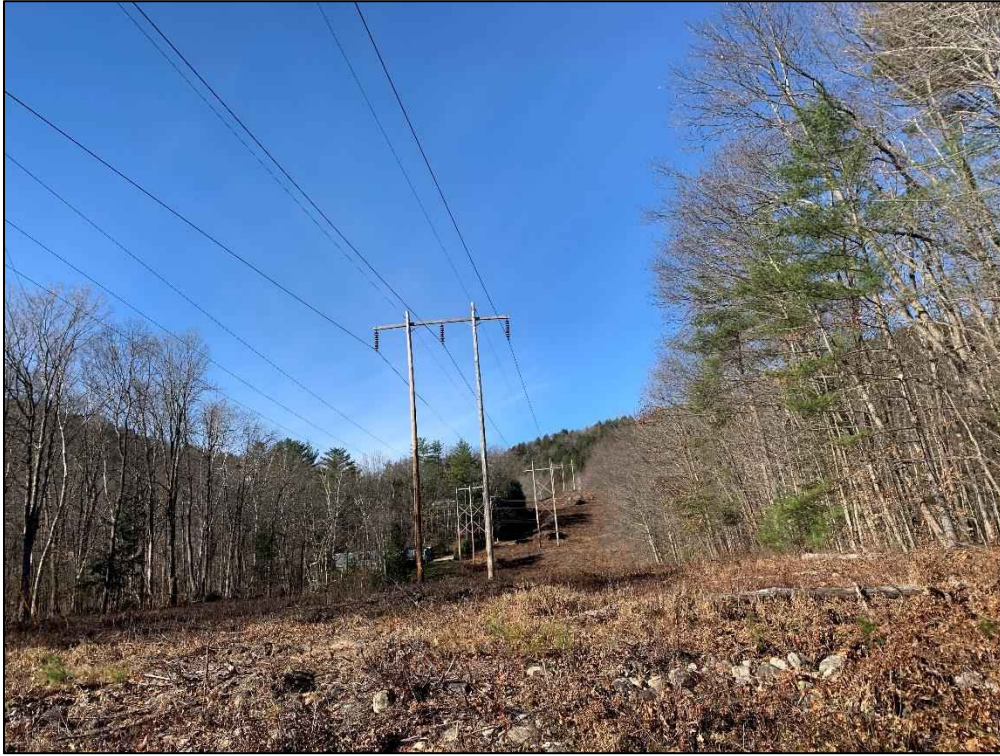
Photograph No. 5: Looking easterly at proposed access toward Structure 174.
