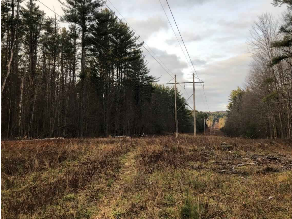
Photograph No. 69: Looking northerly at proposed access toward Structure 364.
