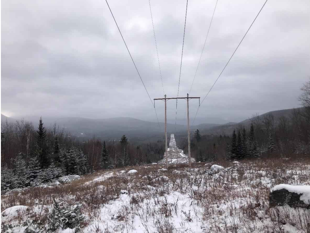
Photograph No. 27: Looking southerly at proposed access toward Structure 321.
