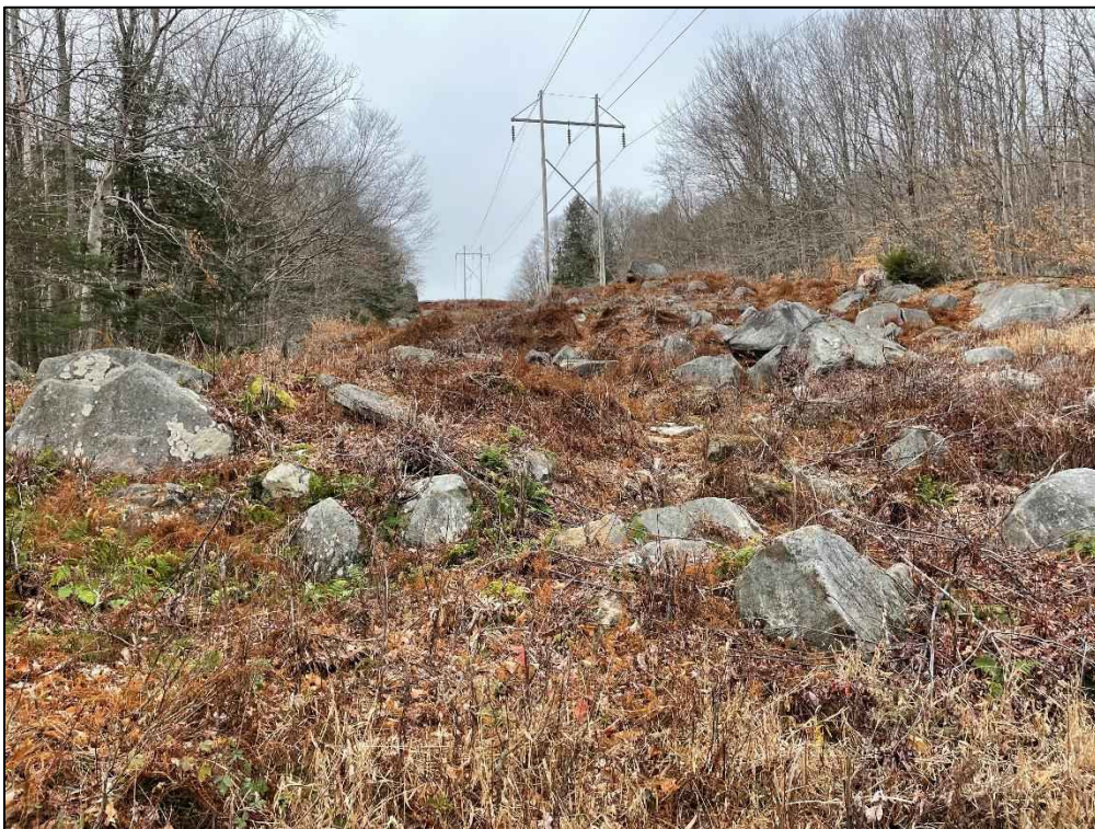
Photograph No. 10: Looking easterly at proposed access toward Structure 179.
