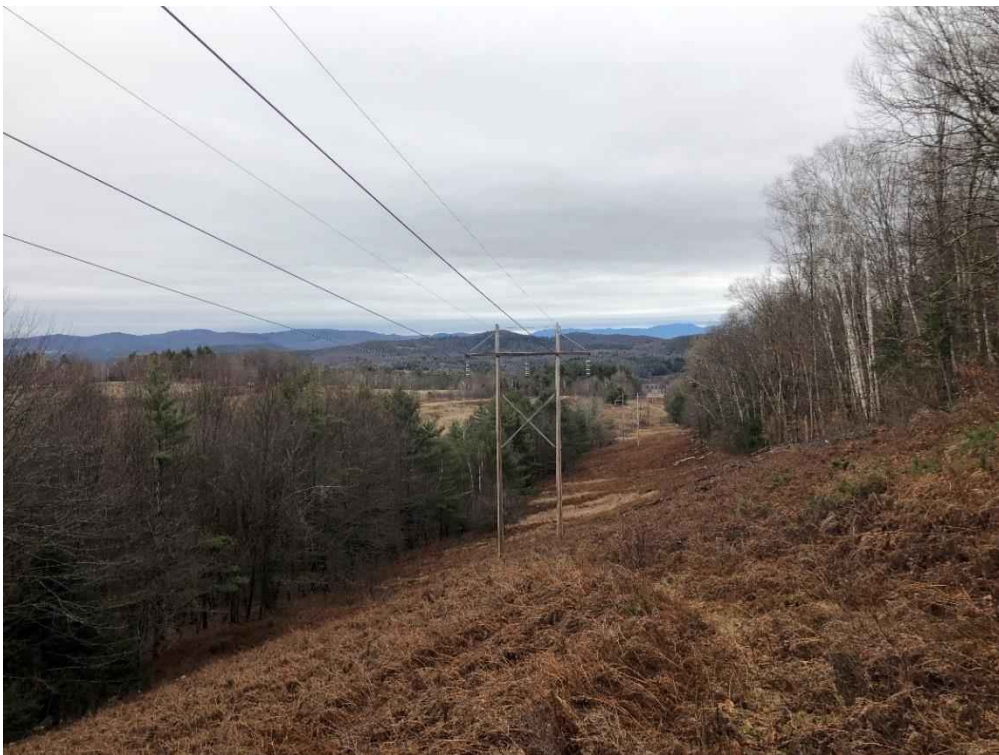
Photograph No. 92: Looking northeasterly at proposed access toward Structure 386.
