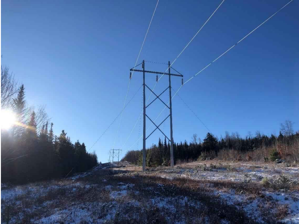
Photograph No. 45: Looking southerly at proposed access toward Structure 339.
