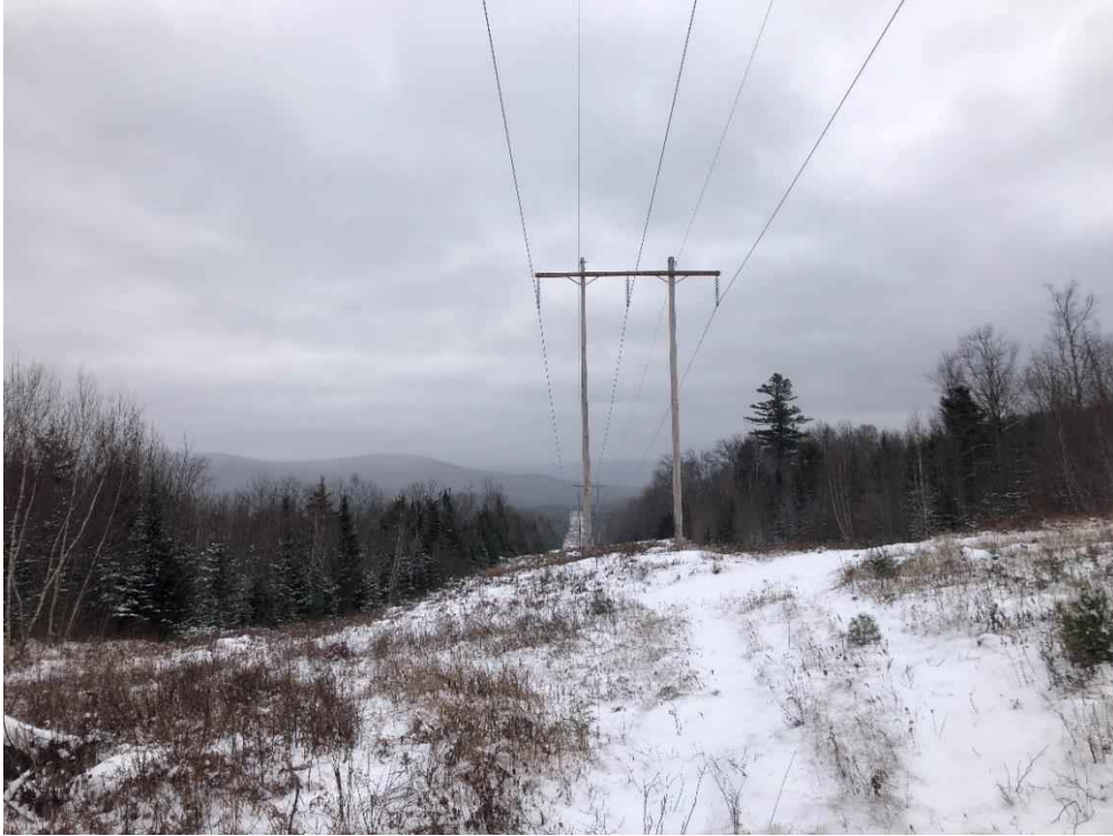
Photograph No. 25: Looking southerly at proposed access toward Structure 319.
