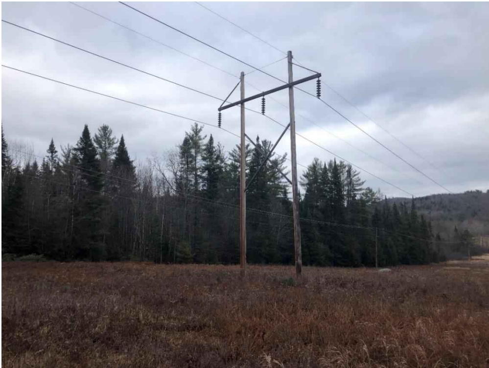
Photograph No. 104: Looking northeasterly at proposed access and work pad location for Structure 398.
