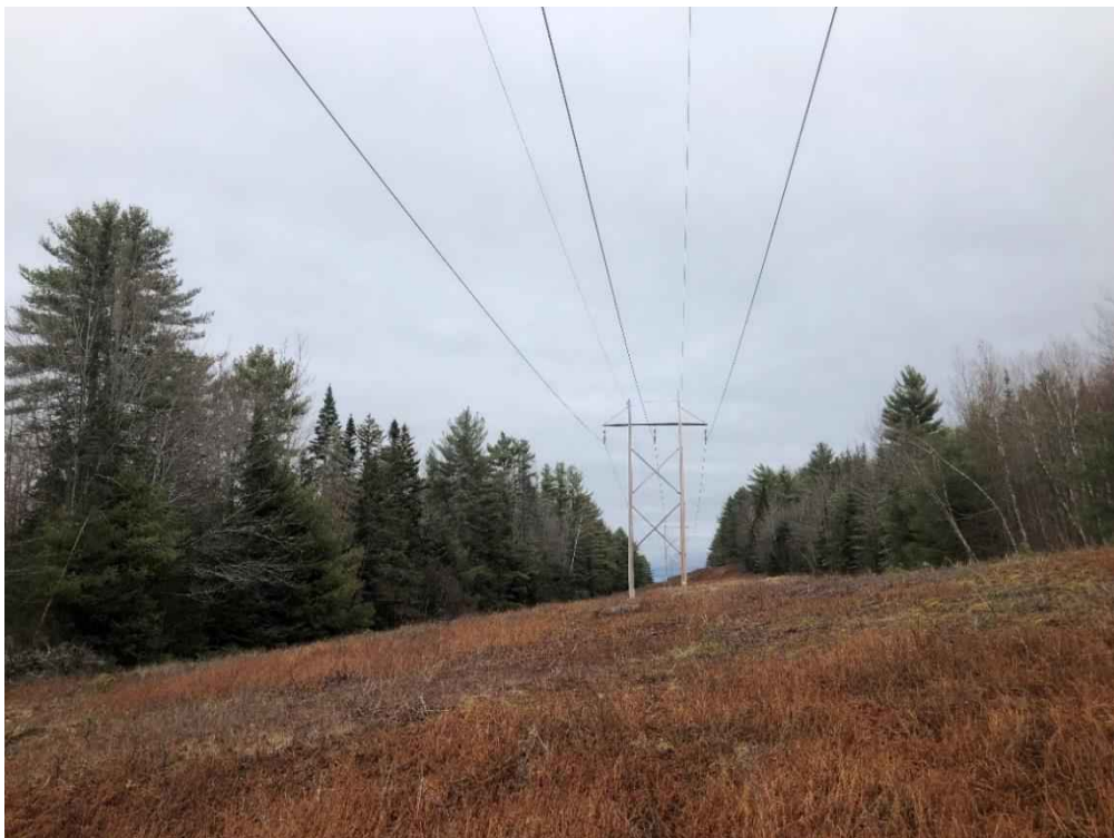
Photograph No. 88: Looking northeasterly at proposed access toward Structure 382.
