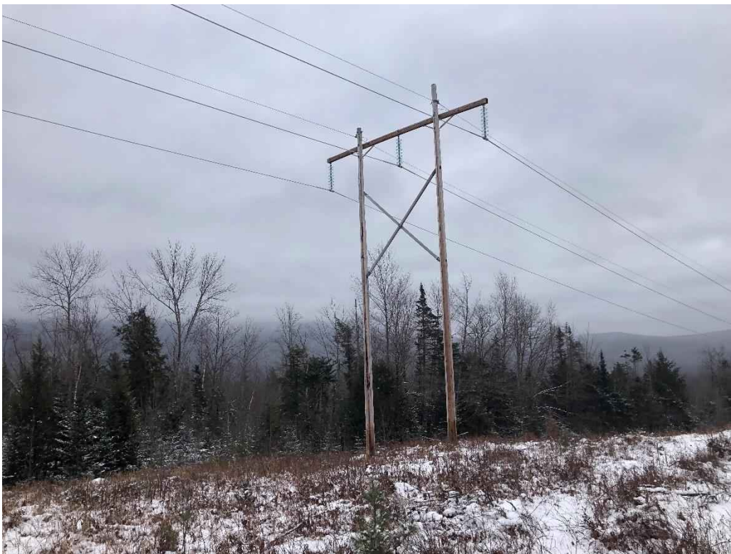
Photograph No. 24: Looking southerly at proposed access and work pad location for Structure 318.
