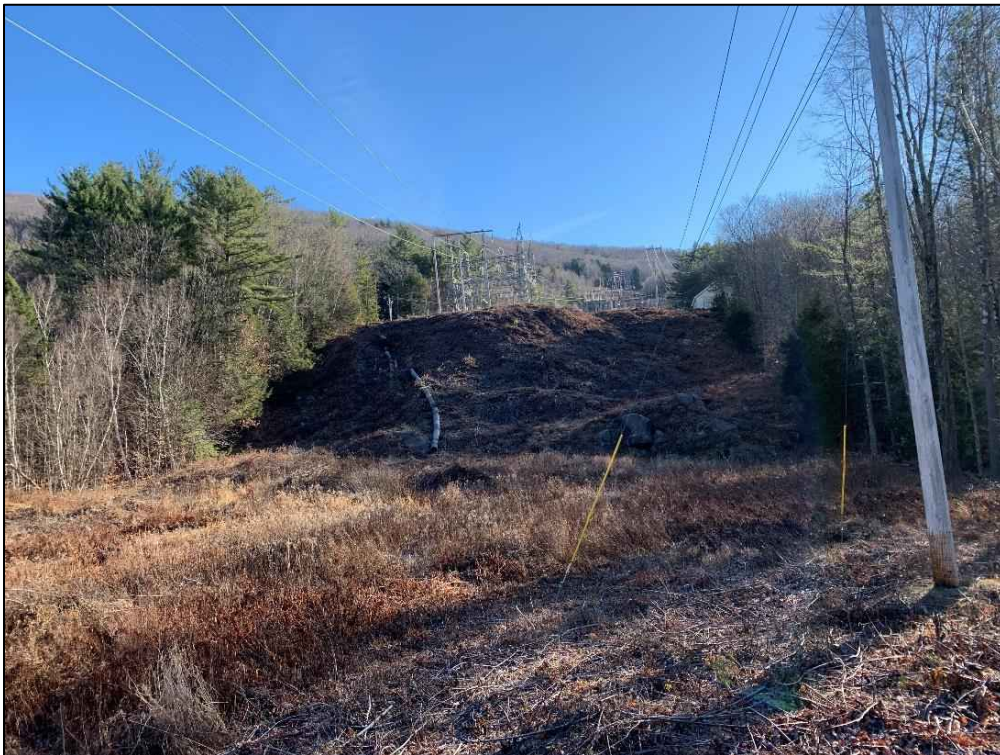
Photograph No. 2: Looking easterly at proposed access and work pad location for Structure 171.
