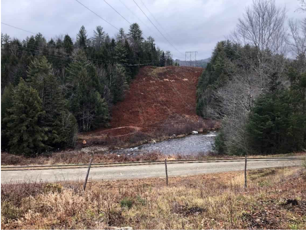
Photograph No. 103: Looking northeasterly toward Structure 397.
