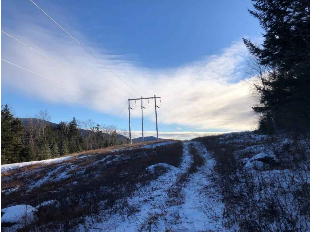
Photograph No. 31: Looking southerly at proposed access toward Structure 325.
