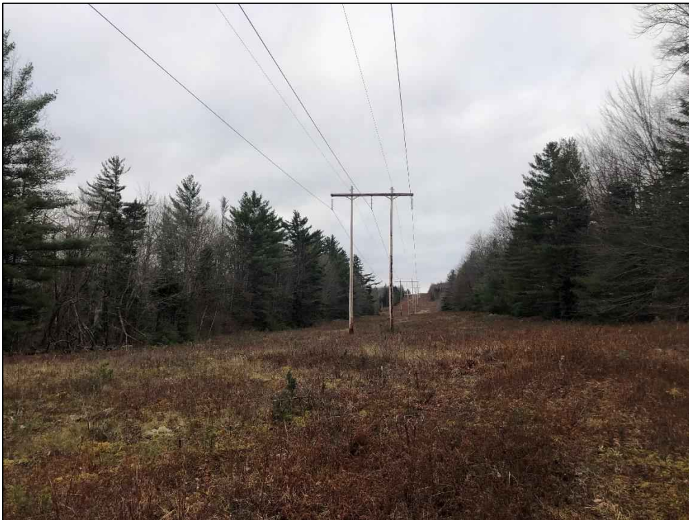
Photograph No. 48: Looking northerly at proposed access toward Structure 342.
