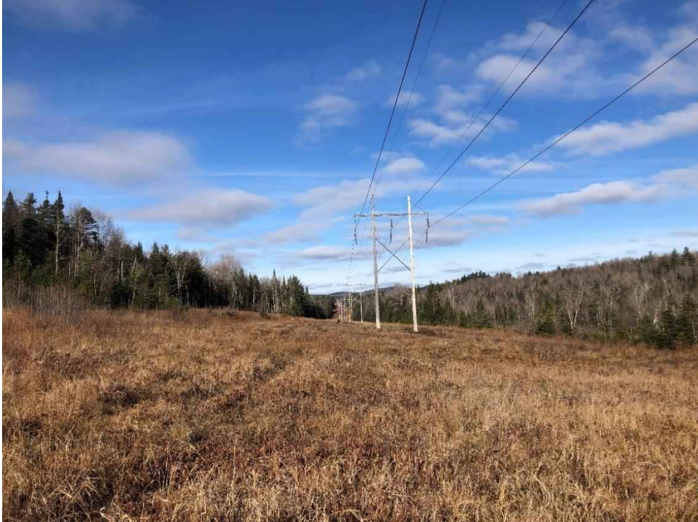
Photograph No. 55: Looking northerly at proposed access toward Structure 350.
