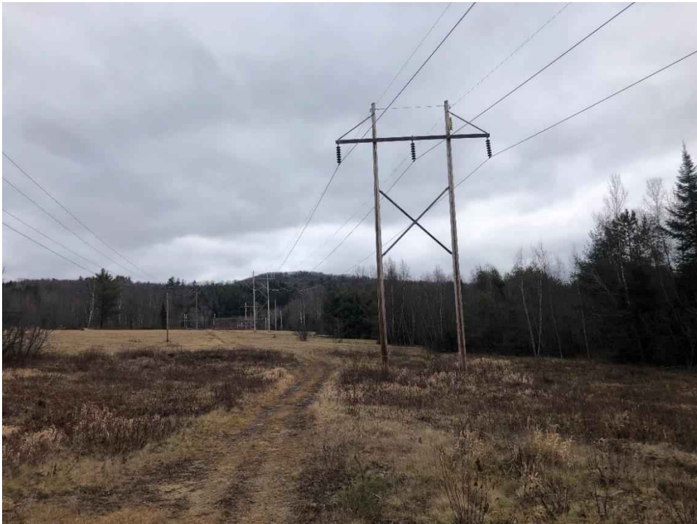
Photograph No. 106: Looking northeasterly at proposed access and work pad location for Structure 400.
