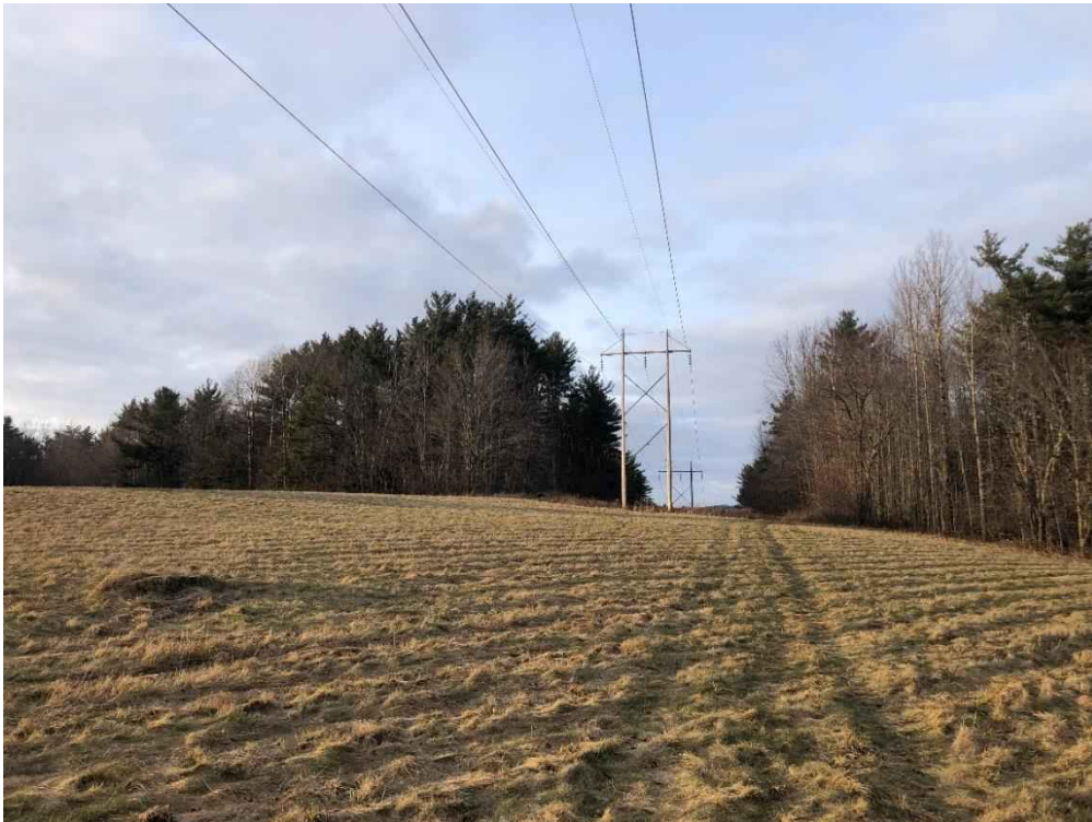
Photograph No. 68: Looking northerly at proposed access toward Structure 363.
