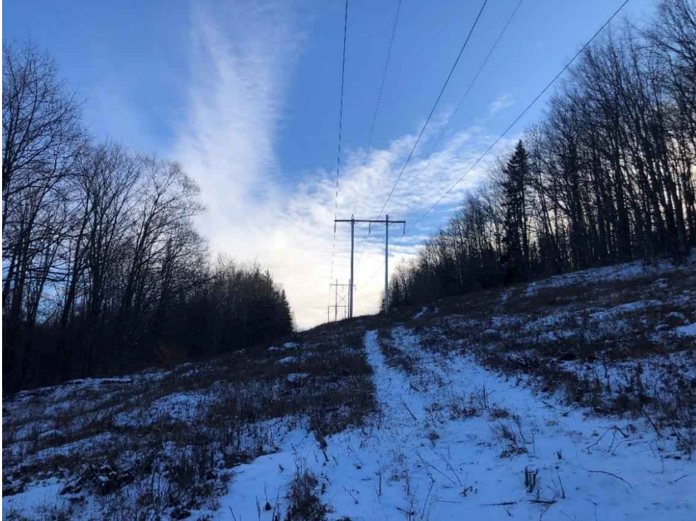
Photograph No. 33: Looking southerly at proposed access toward Structure 327.
