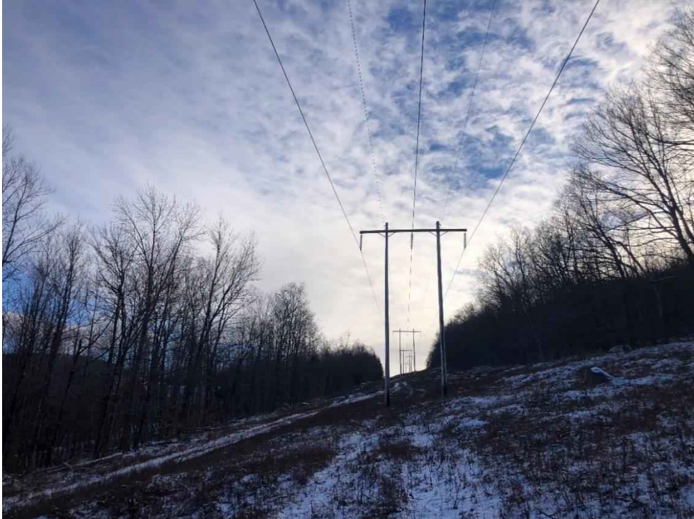
Photograph No. 35: Looking southerly at proposed access toward Structure 329.
