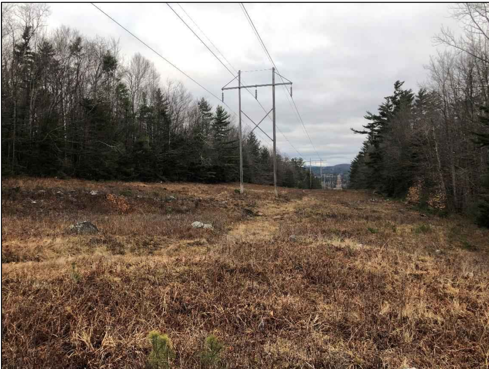
Photograph No. 46: Looking northerly at proposed access toward Structure 340.
