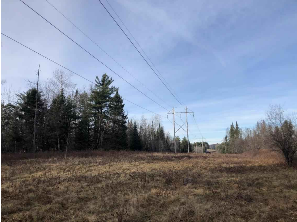
Photograph No. 63: Looking northerly at proposed access toward Structure 358.
