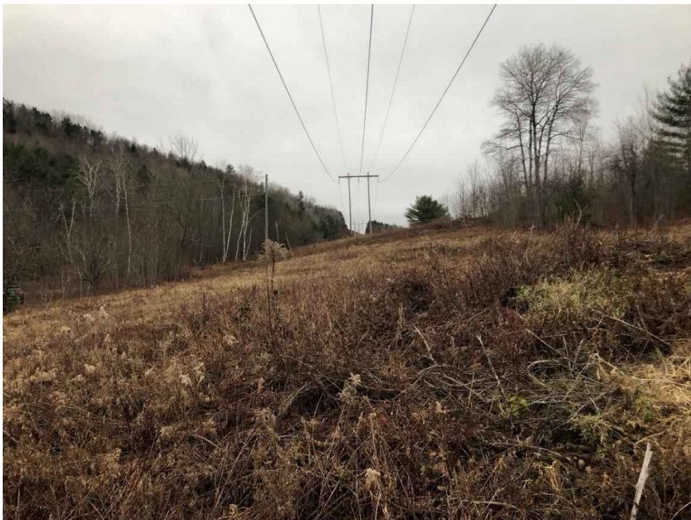
Photograph No. 96: Looking northeasterly at proposed access toward Structure 390.
