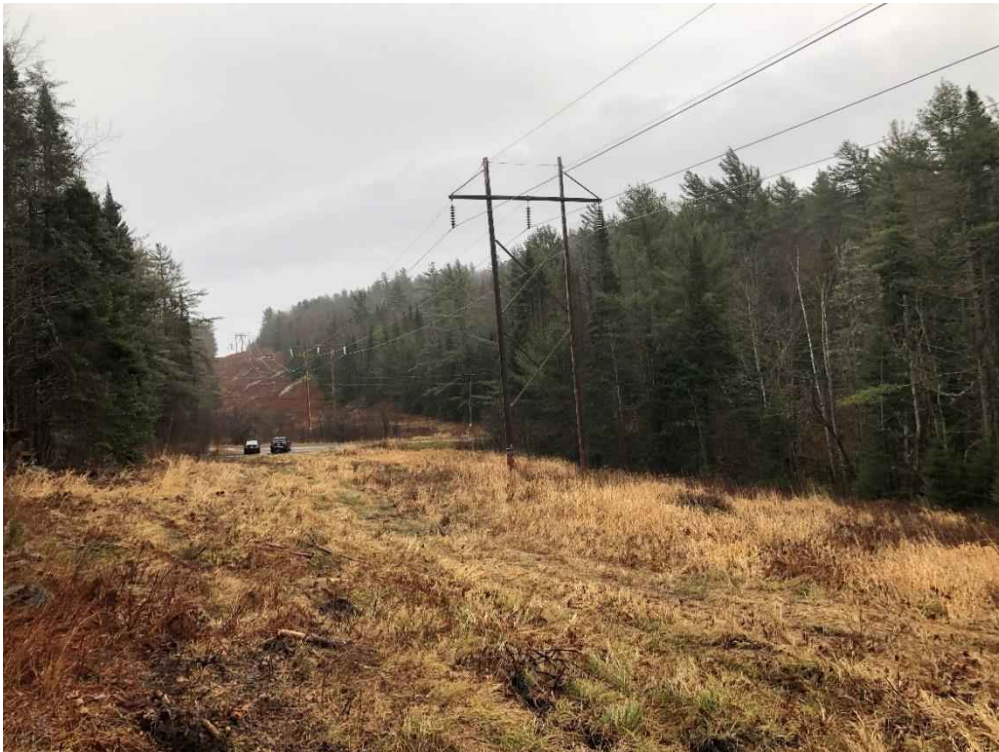
Photograph No. 80: Looking northeasterly at proposed access toward Structure 375.
