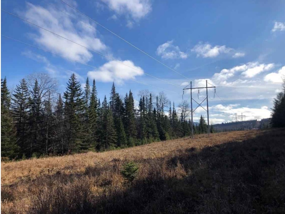
Photograph No. 57: Looking southerly at proposed access toward Structure 352.
