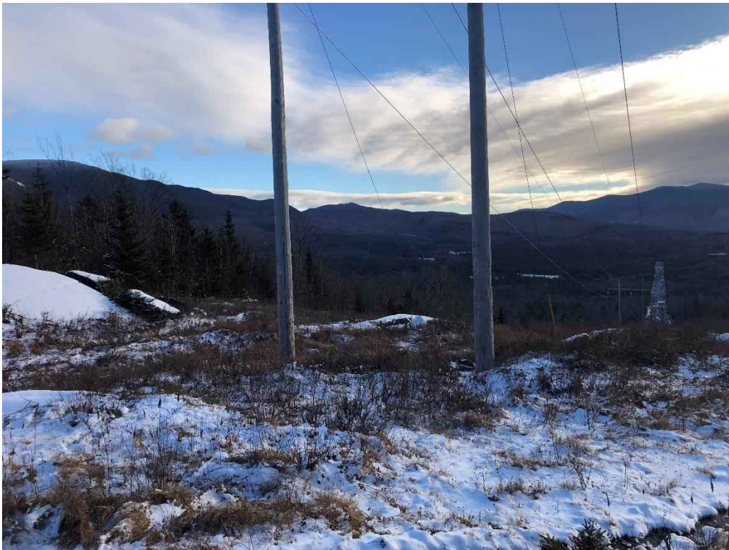
Photograph No. 30: Looking southerly at proposed work pad location for Structure 324.
