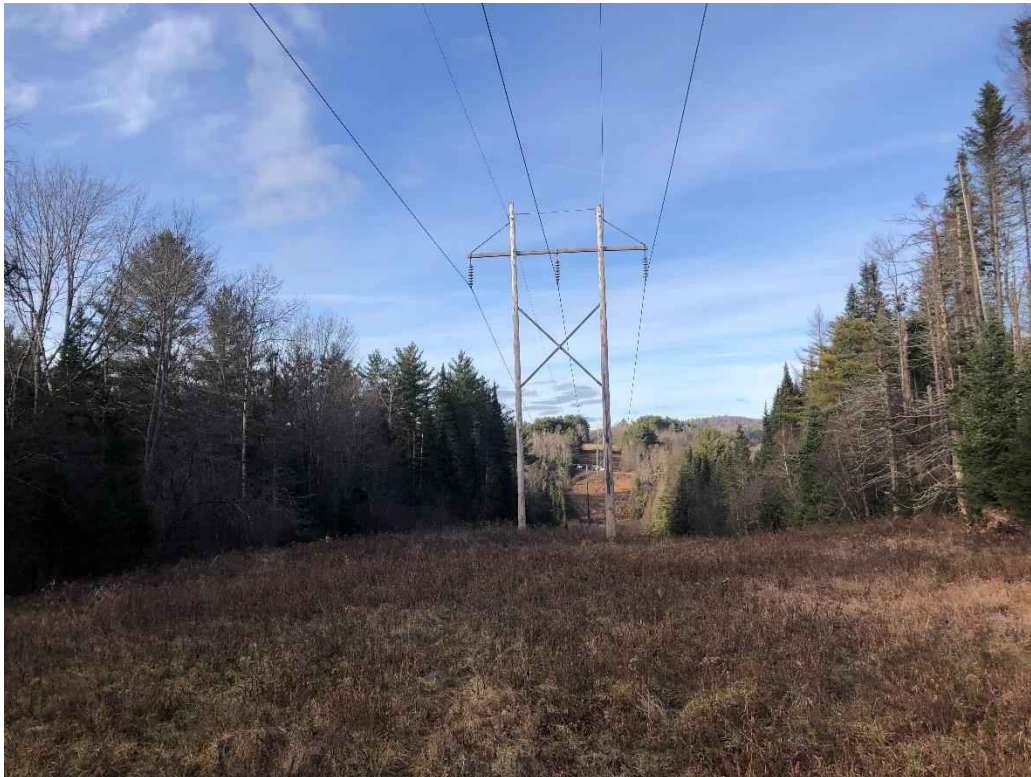
Photograph No. 64: Looking northerly at proposed access toward Structure 359.
