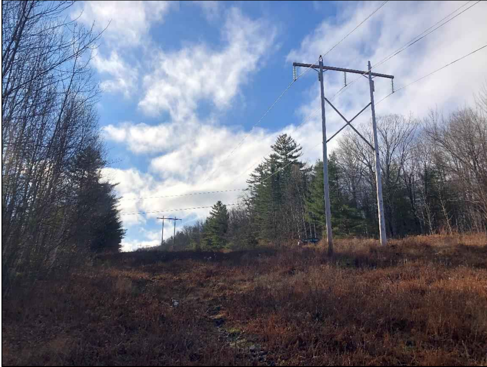
Photograph No. 49: Looking southerly at proposed access and work pad location for Structure 343.
