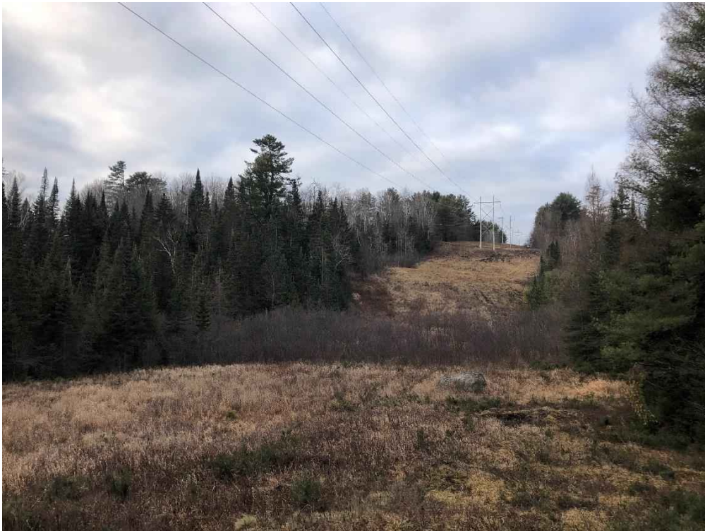
Photograph No. 66: Looking northerly at proposed access toward Structure 361.
