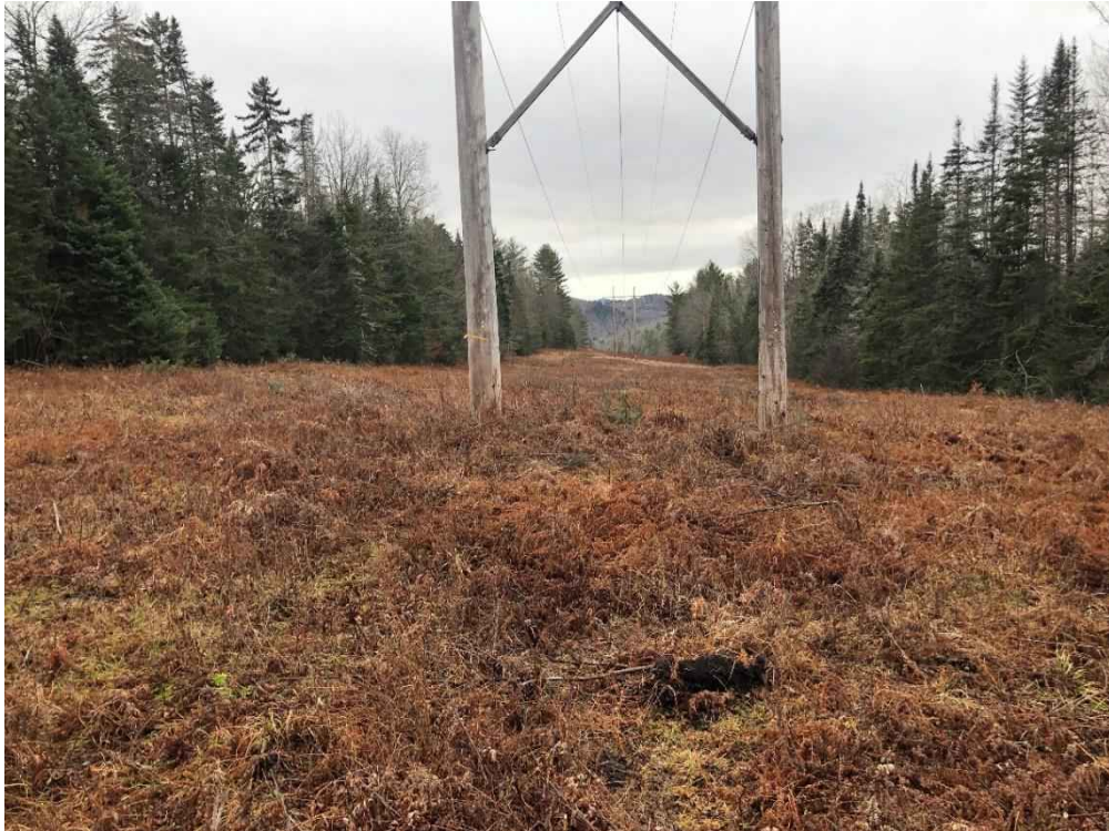
Photograph No. 87: Looking southwestly at proposed work pad location for Structure 381.
