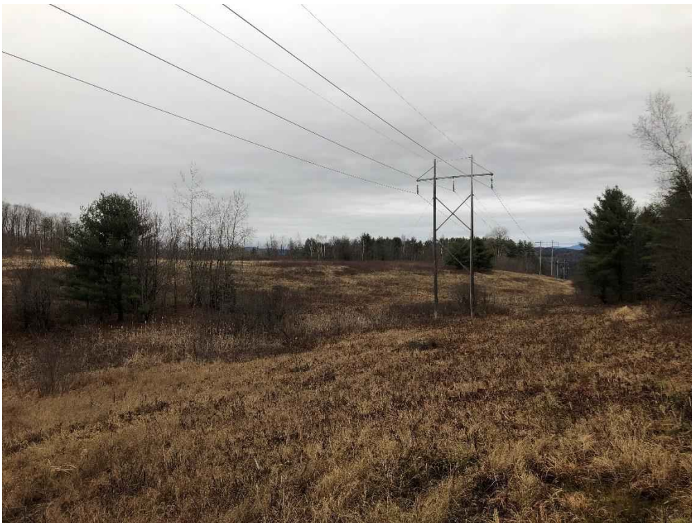
Photograph No. 94: Looking northerly at proposed access toward Structure 388.
