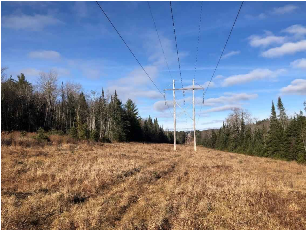
Photograph No. 56: Looking northerly at proposed access toward Structure 351.
