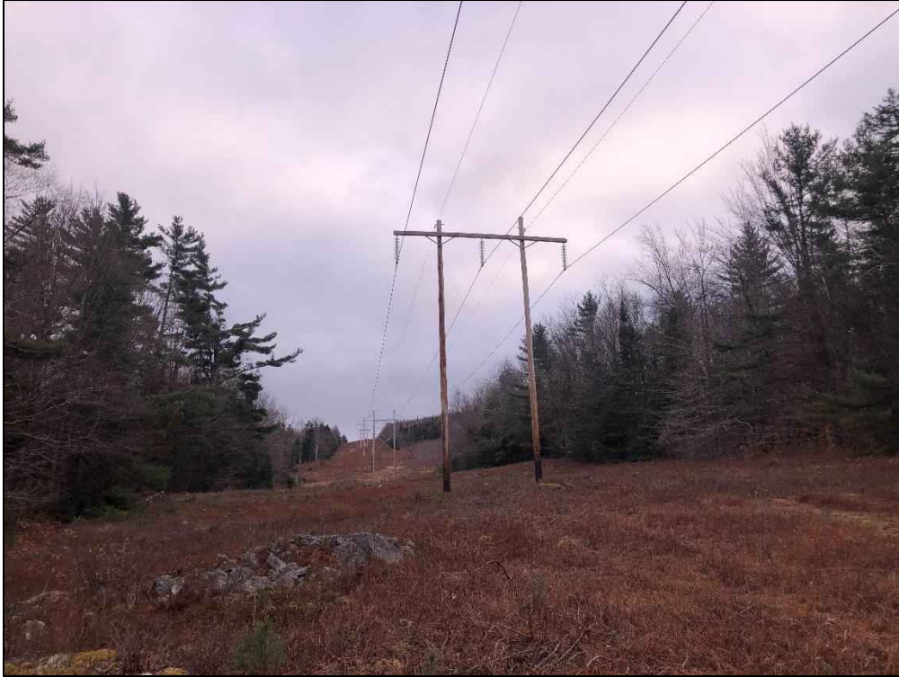
Photograph No. 47: Looking northerly at proposed access toward Structure 341.
