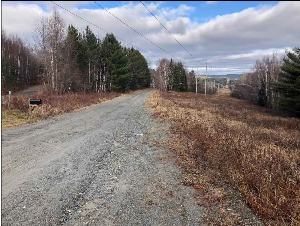
Photograph No. 51: Looking northwesterly at proposed access toward Structure 345 from Presley Road.
