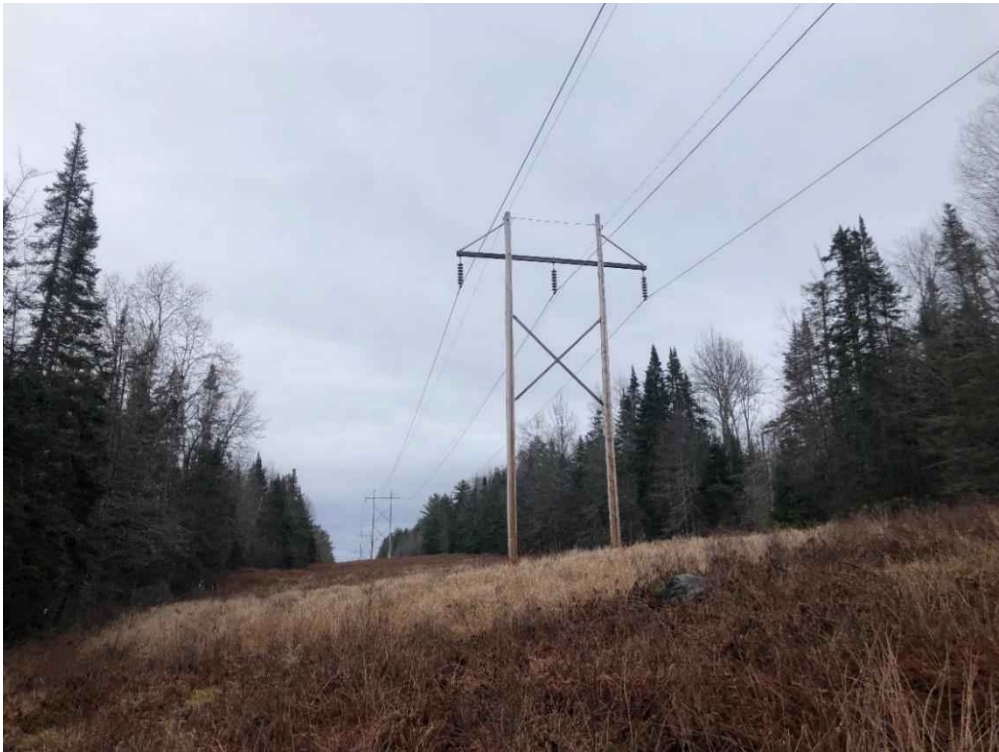
Photograph No. 86: Looking northeasterly at proposed access toward Structure 380.
