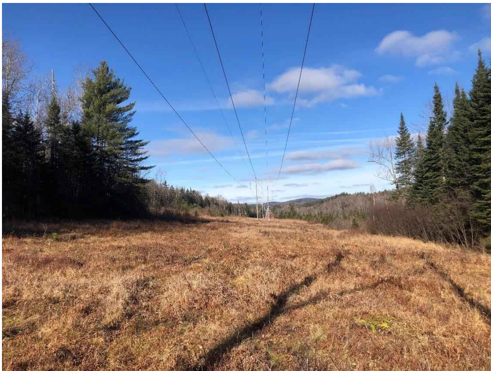
Photograph No. 54: Looking northerly at proposed access toward Structure 349.
