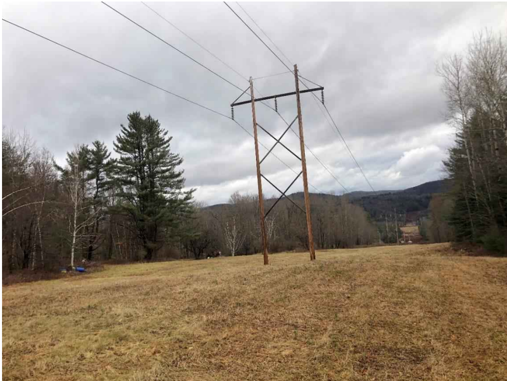
Photograph No. 98: Looking northeasterly at proposed access and work pad location for Structure 392.
