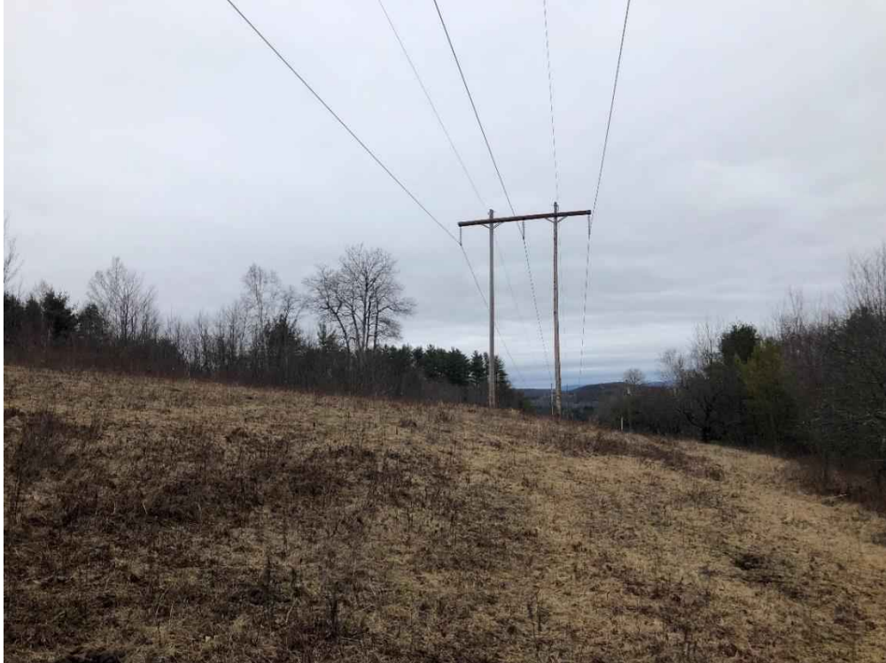
Photograph No. 95: Looking northeasterly at proposed access toward Structure 389.
