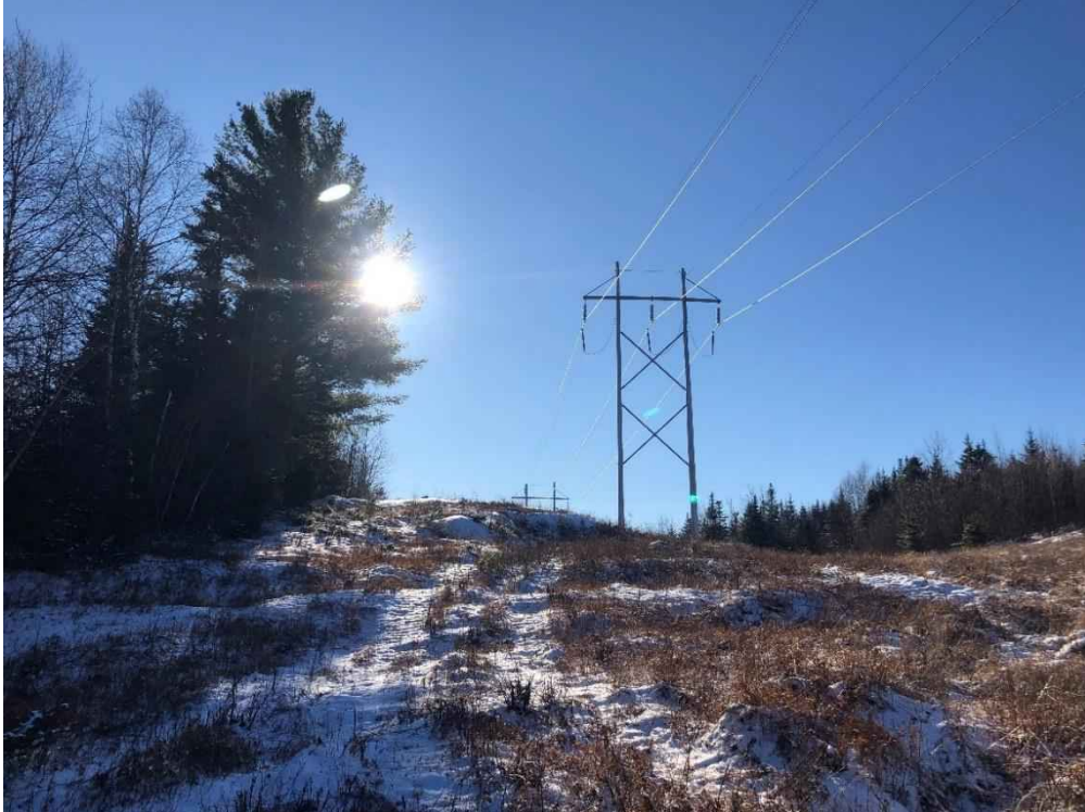
Photograph No. 41: Looking southerly at proposed access toward Structure 335.
