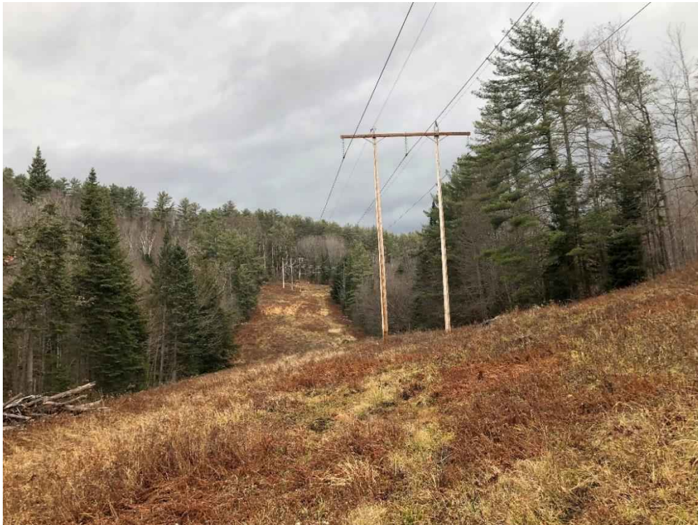
Photograph No. 78: Looking northerly at proposed access toward Structure 373.
