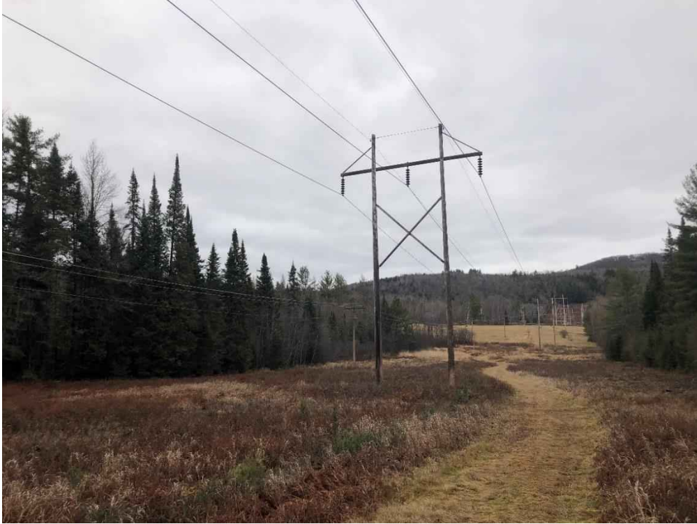
Photograph No. 105: Looking northeasterly at proposed access and work pad location for Structure 399.
