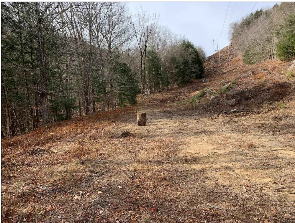
Photograph No. 8: Looking easterly at proposed access toward Structure 177.
