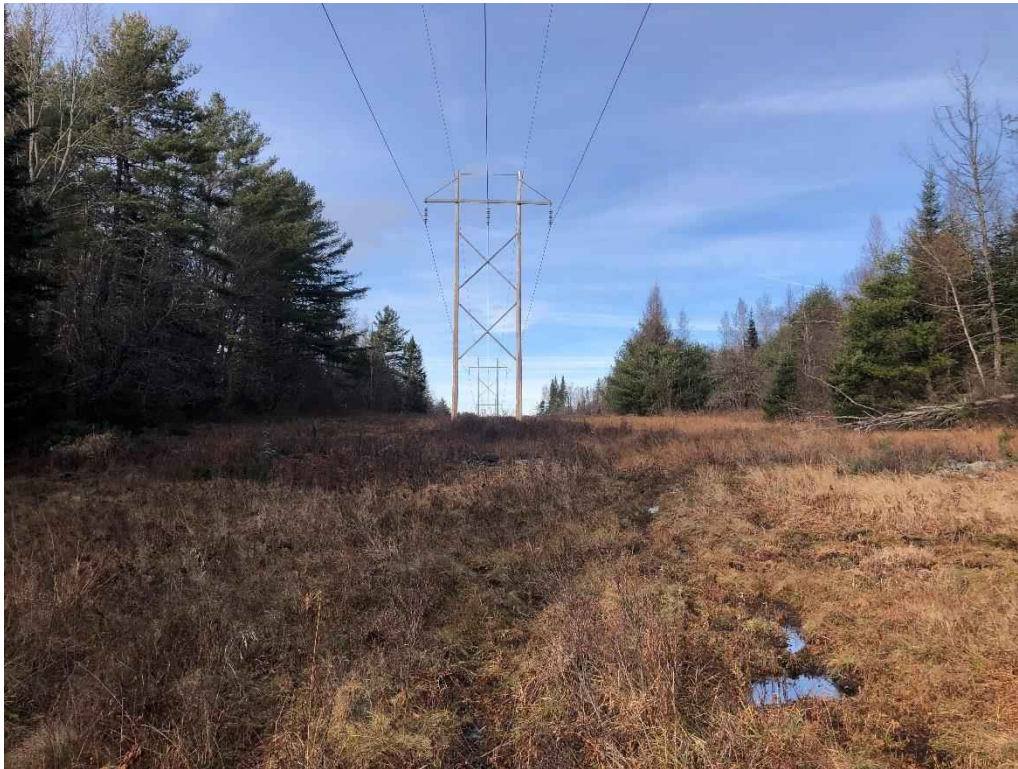
Photograph No. 62: Looking northerly at proposed access toward Structure 357.
