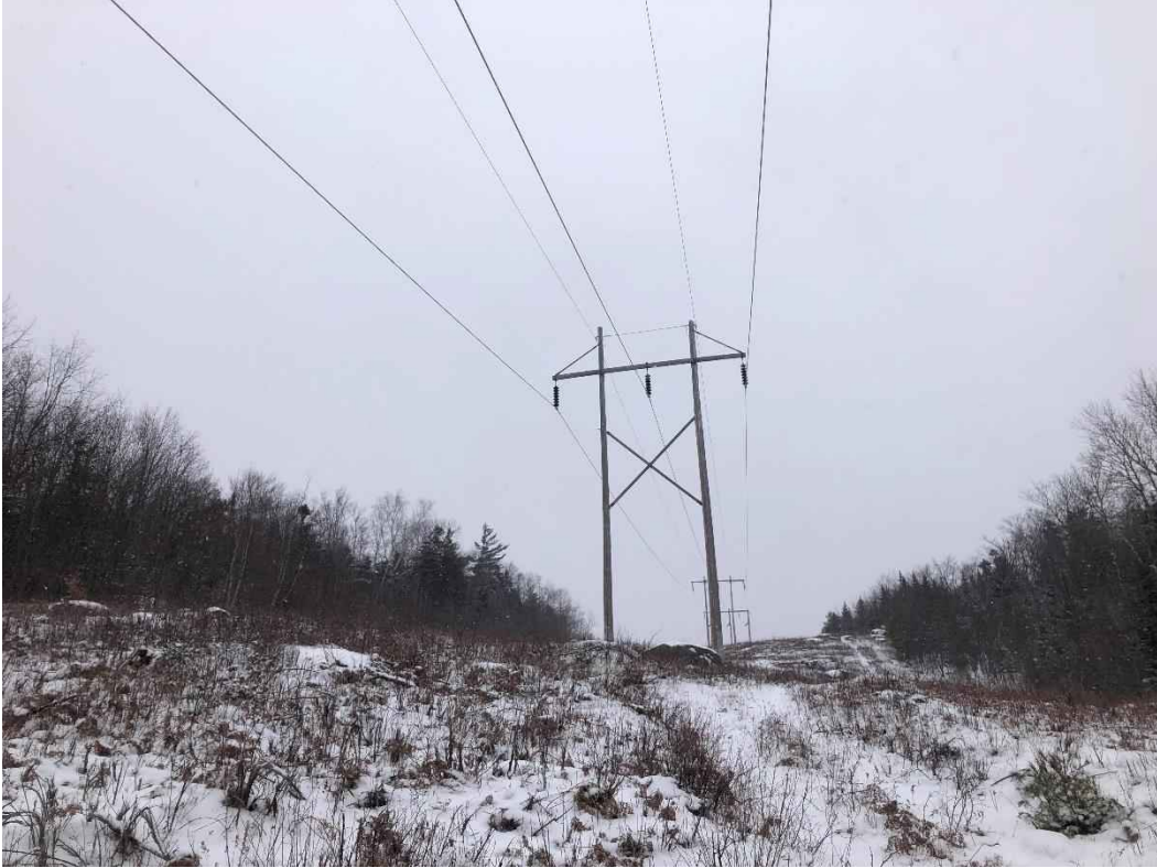
Photograph No. 29: Looking southerly at proposed access toward Structure 323.
