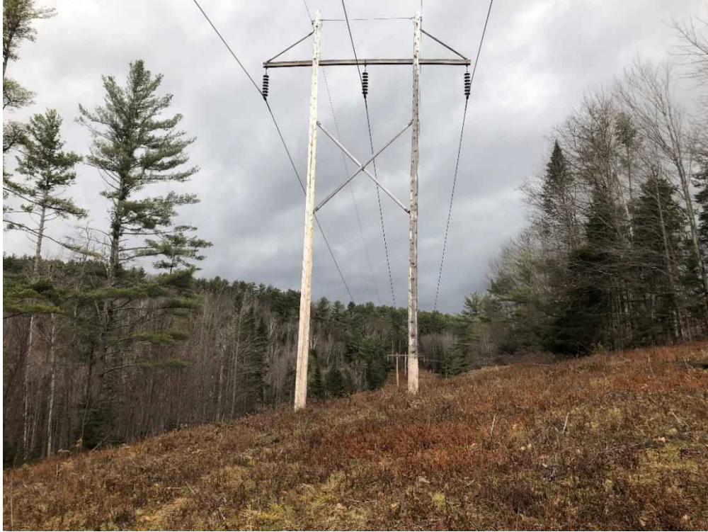
Photograph No. 77: Looking northerly at proposed access and work pad location for Structure 372.
