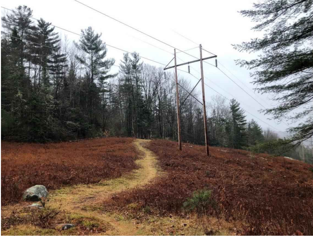
Photograph No. 85: Looking northwesterly at proposed access toward Structure 379.
