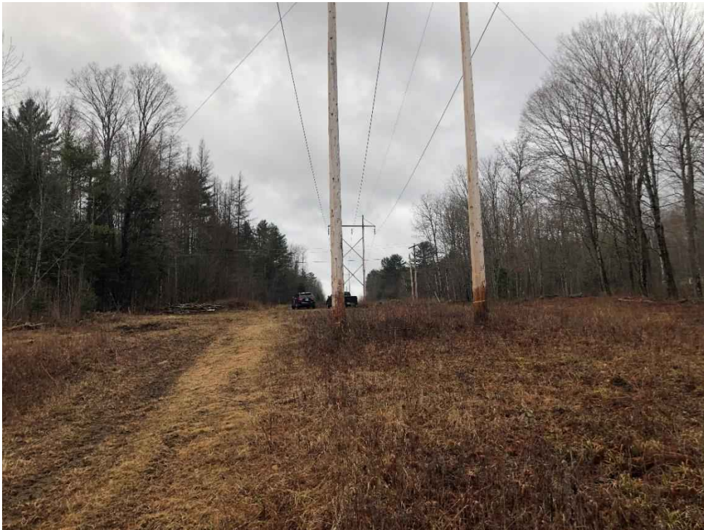
Photograph No. 100: Looking southwesterly at proposed work pad location for Structure 394.
