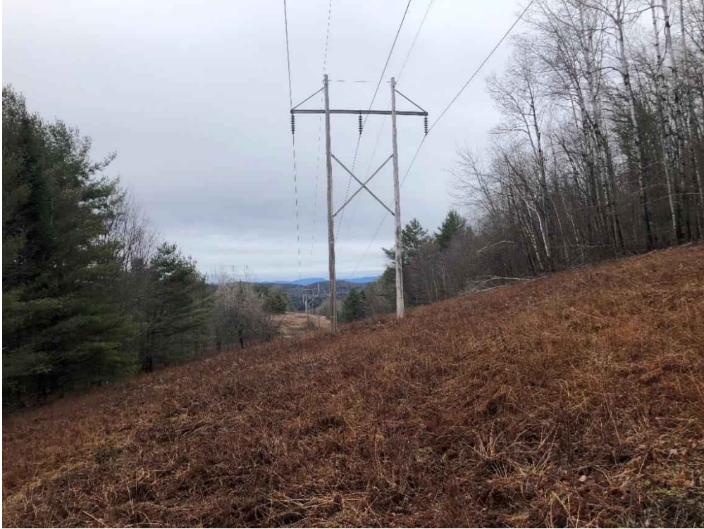
Photograph No. 93: Looking northeasterly at proposed access toward Structure 387.
