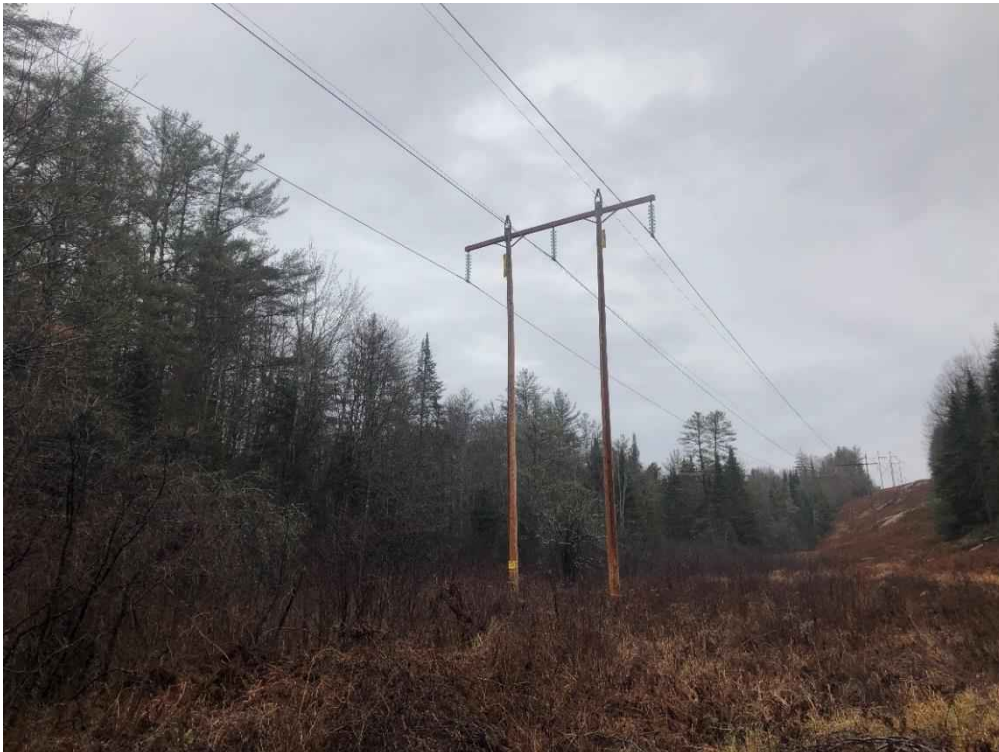
Photograph No. 82: Looking northerly at proposed access and work pad location for Structure 376.
