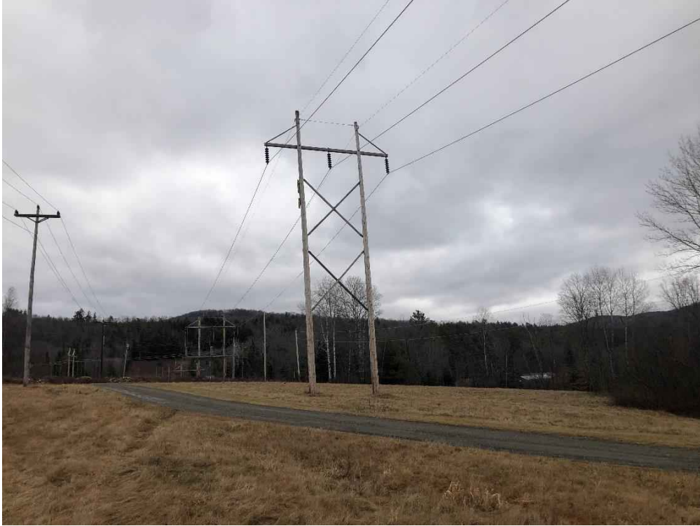
Photograph No. 107: Looking northeasterly at proposed access toward Structure 401.
