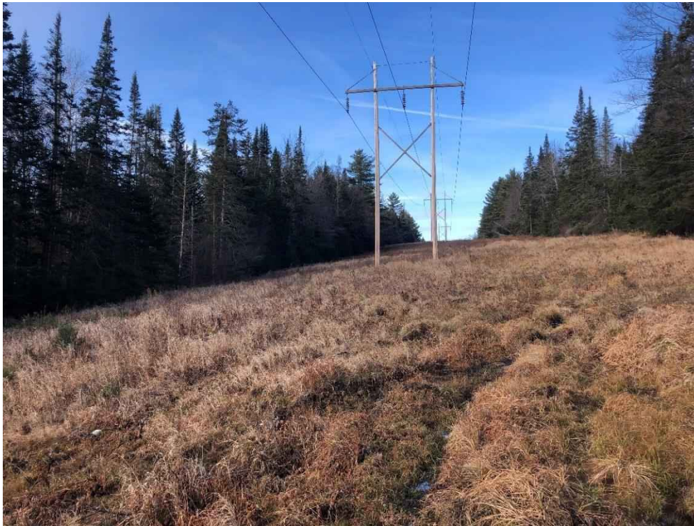
Photograph No. 60: Looking northerly at proposed access toward Structure 355.
