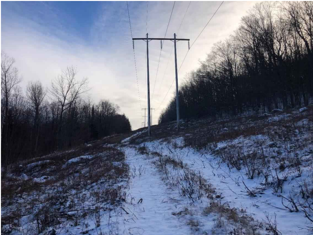
Photograph No. 34: Looking southerly at proposed access toward Structure 328.
