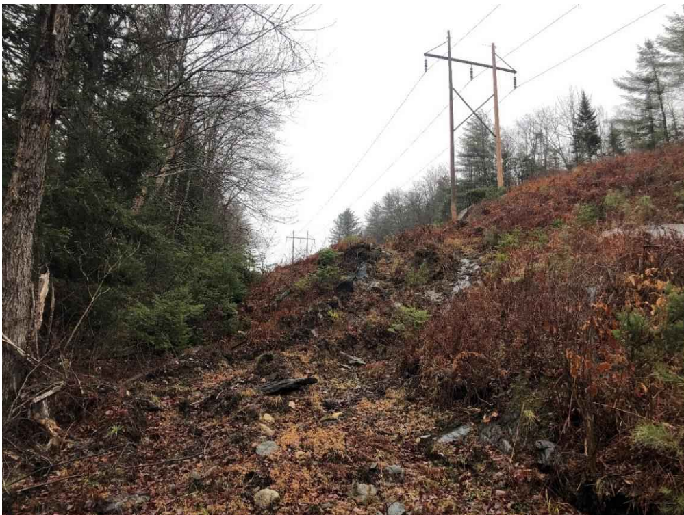
Photograph No. 84: Looking northerly at proposed access toward Structure 378.
