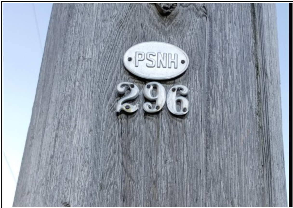
Pole on the Beebe River to Streeter Pond tap (1986) section of the X-178:
