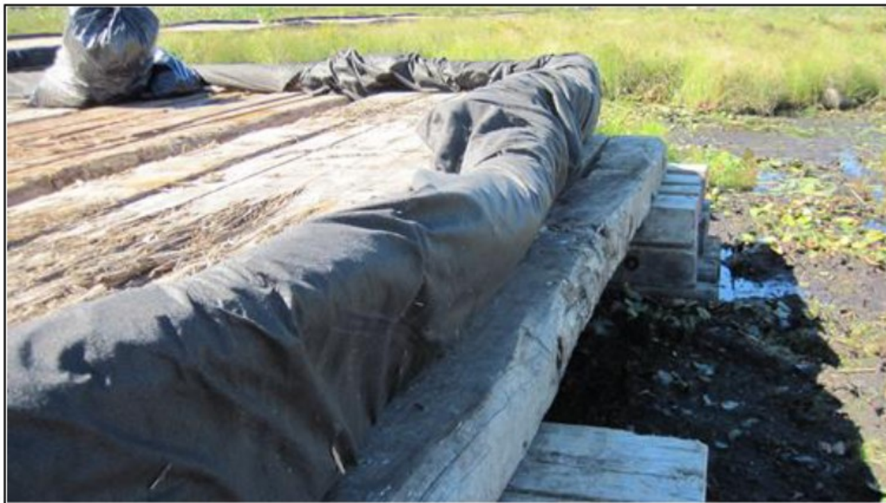
Constructing a swamp mat bridge span reduces direct impacts to the wetland surface and maintains aquatic organism passage through the construction area. The number of necessary swamp mats may be reduced using this method.
