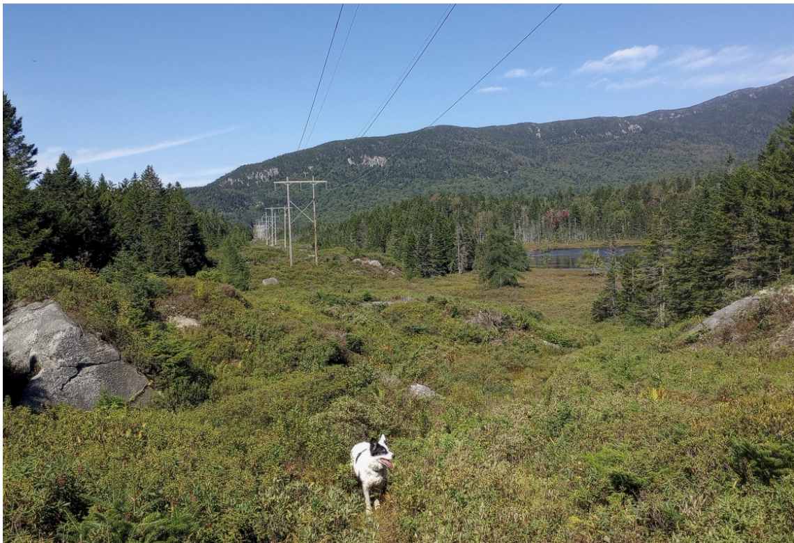
Left: Looking northwest at structure 246/251
