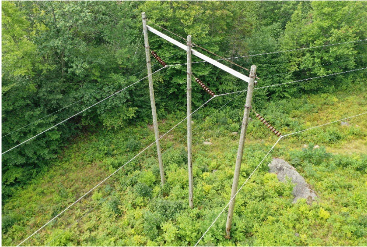
Examples of existing structures to be removed
