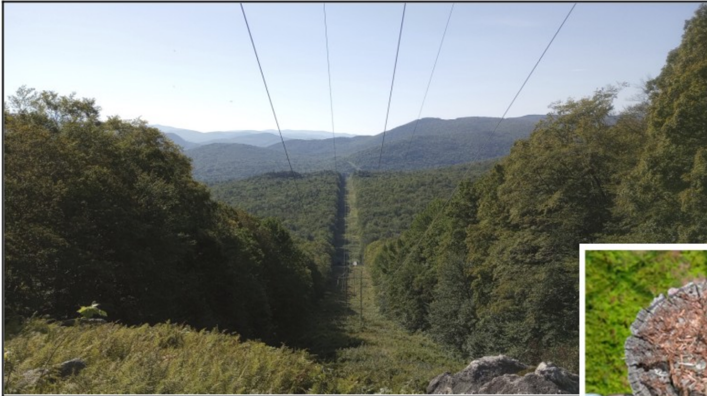
Looking south from structure 211
