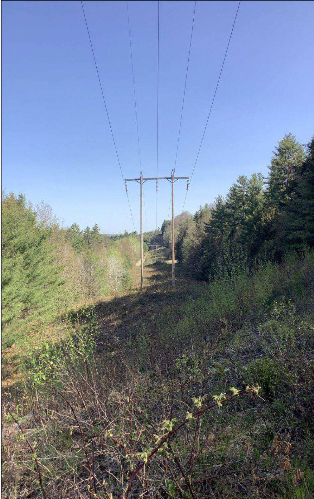
Photo 1: View north away from Huckins Hill Substation.
