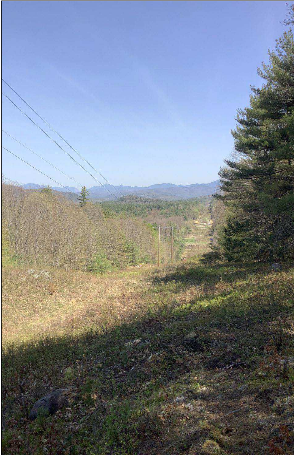
Photo 2: View north near Structure 285 looking down slope towards Structure 286.
