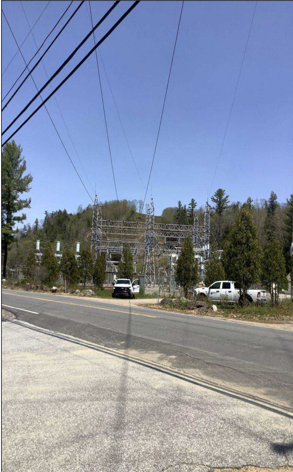
Photo 12: View north at Beebe River Substation
