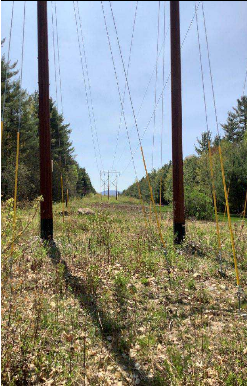
Photo 11: View south along the existing ROW from Beebe River Substation.
