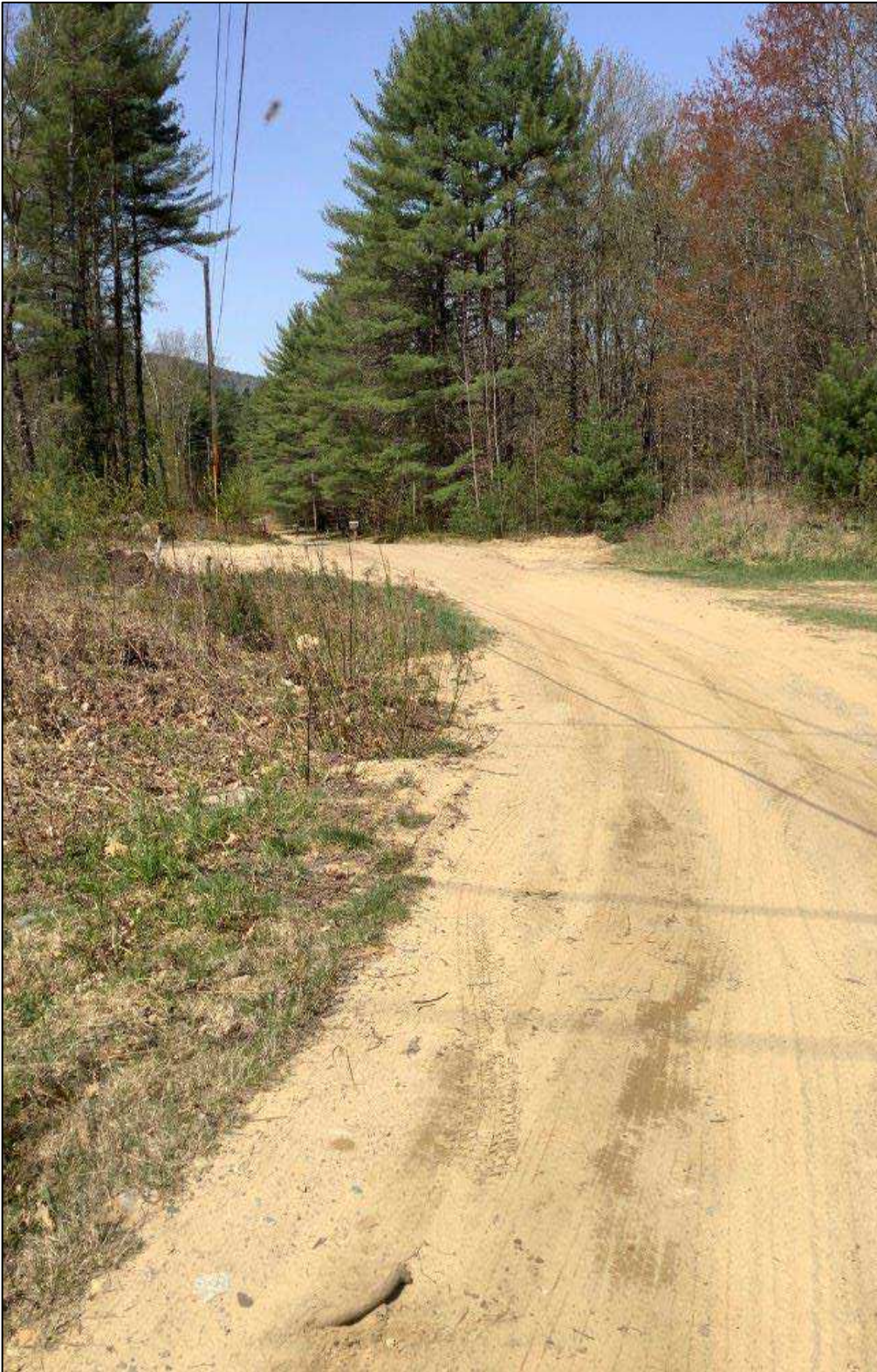
Photo 5: View west of the intersection of Ken Mar Drive and the ROW.
